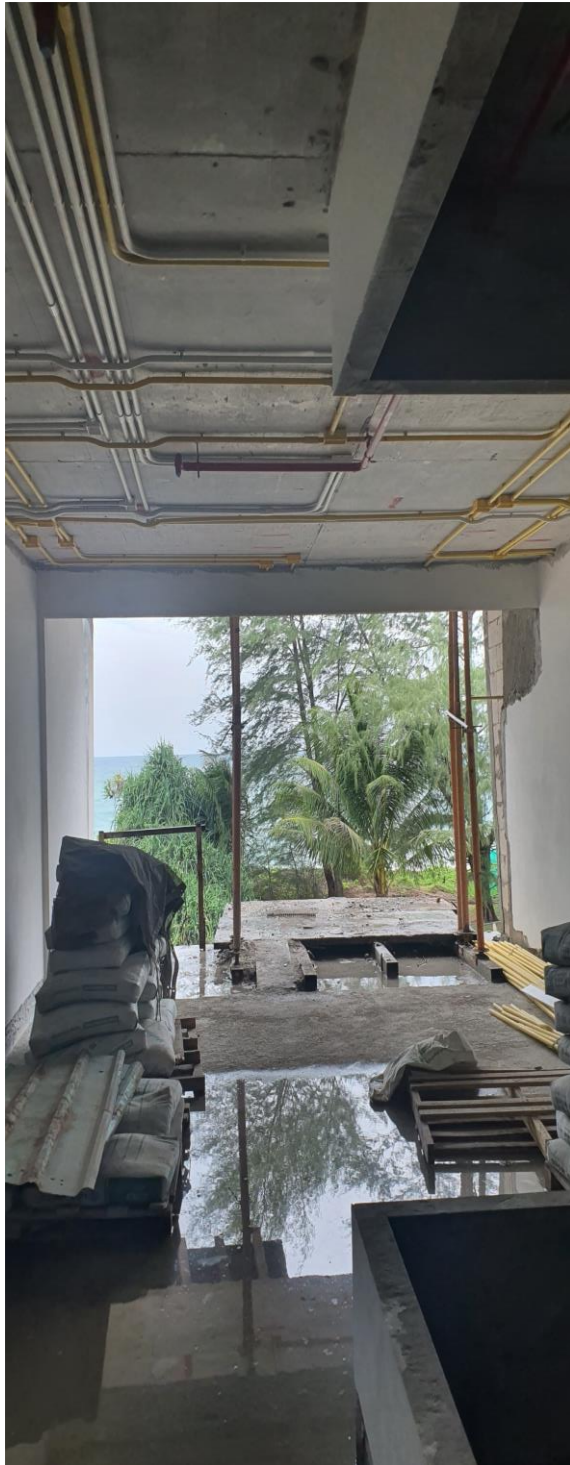
Building 6 Corridor & Rooms, plastering and Conduit works
