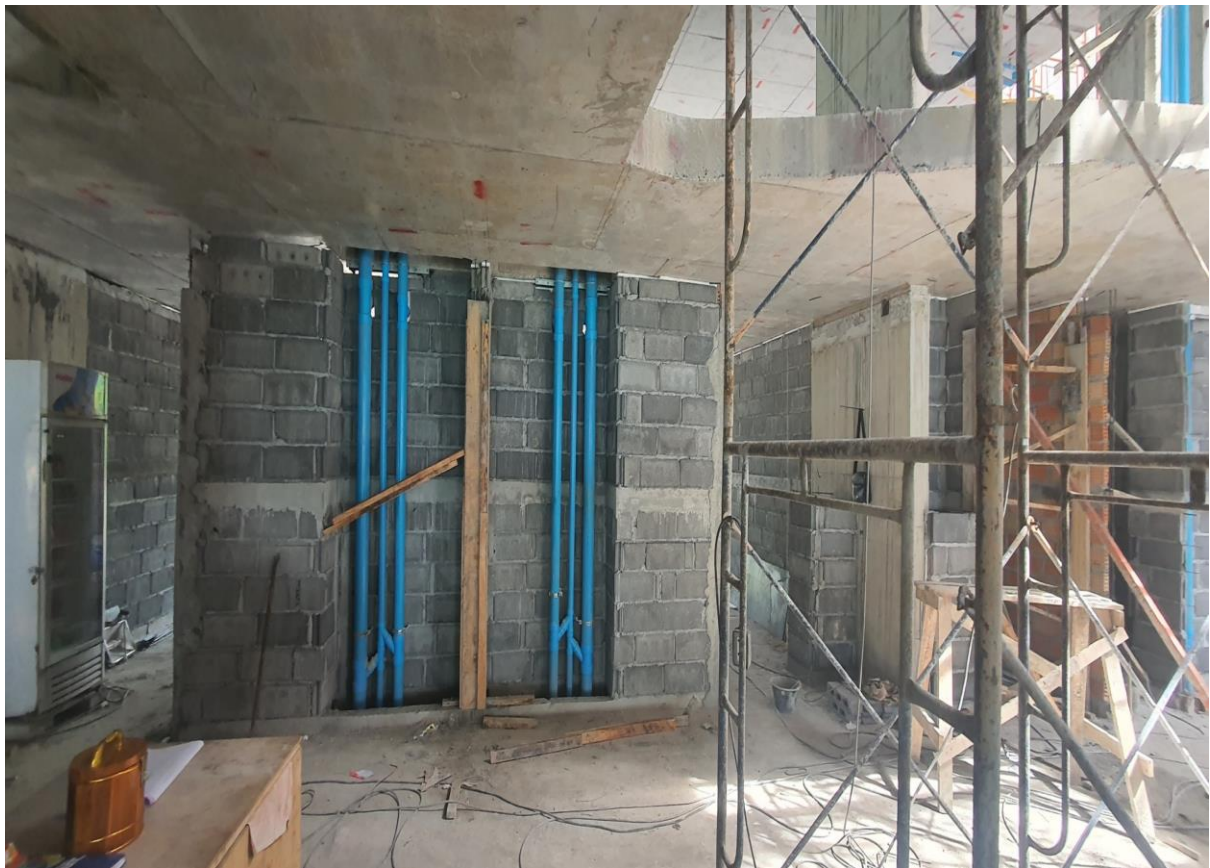
Sleeve and Block work Ground floor Building 1 Units 1006,7,8
