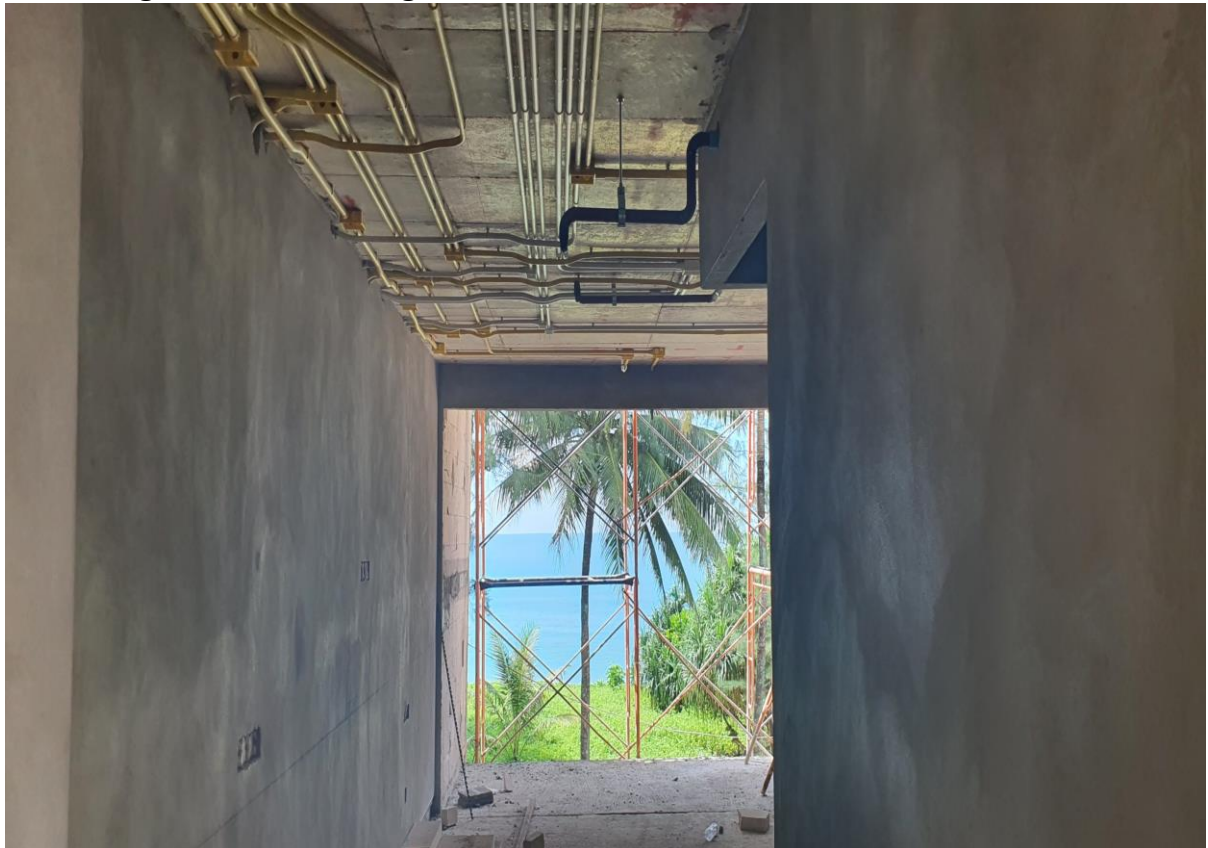
Plastering 1 st Floor Room Building 8 Fire protection pipes visible in room
