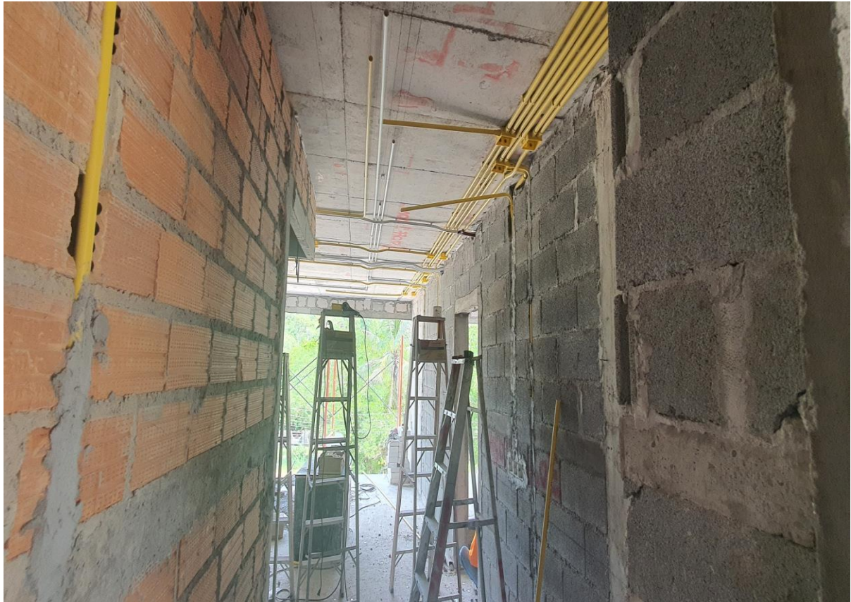
Blockwork and Install Conduit ceiling 1 st Floor Building 4
