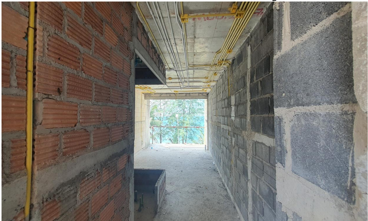
1st Floor Building 2 blockwork/Channel wall conduit work and ceiling conduit work
