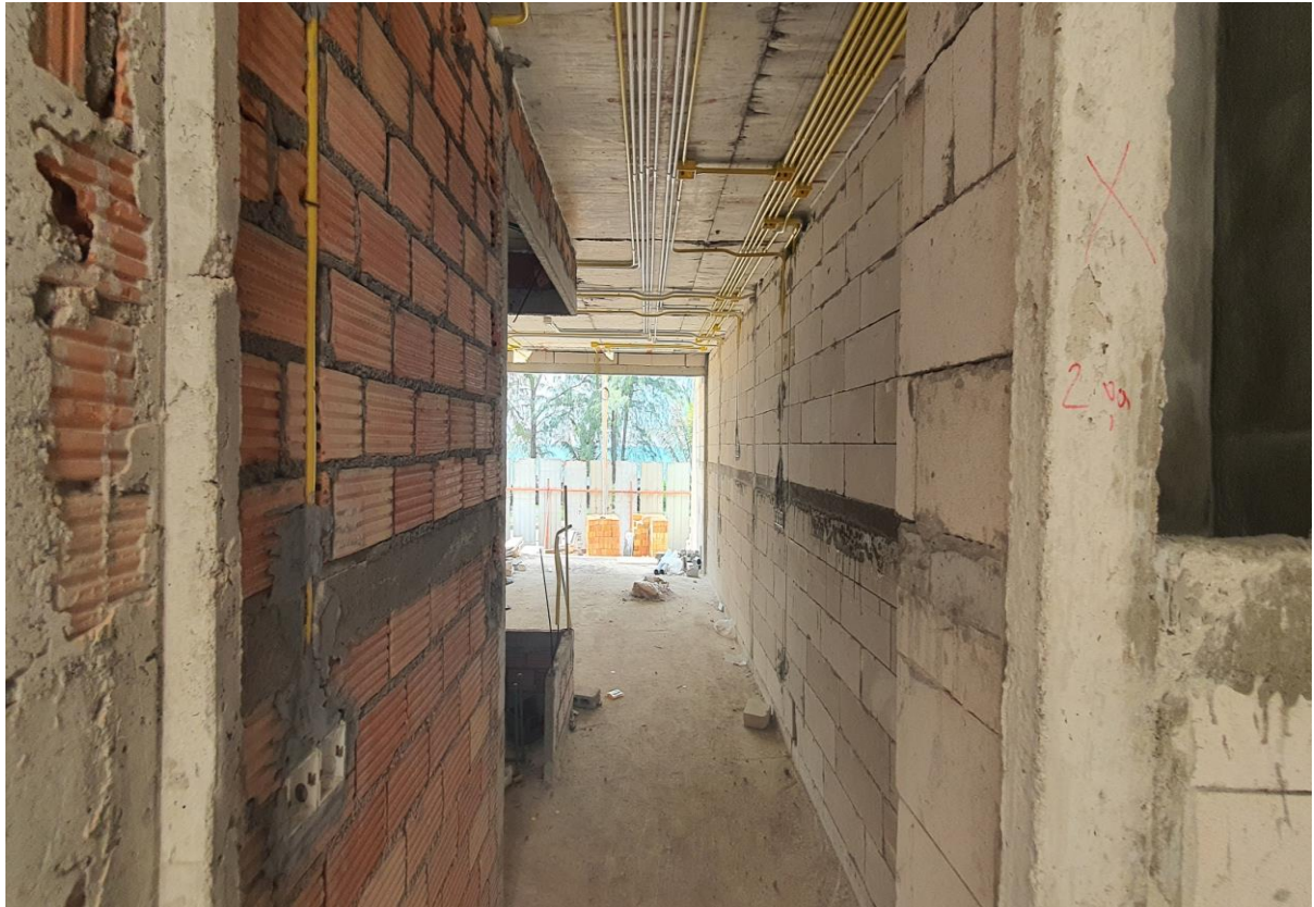
Blockwork /Channel wall Work and ceiling conduit work GF Building 2
