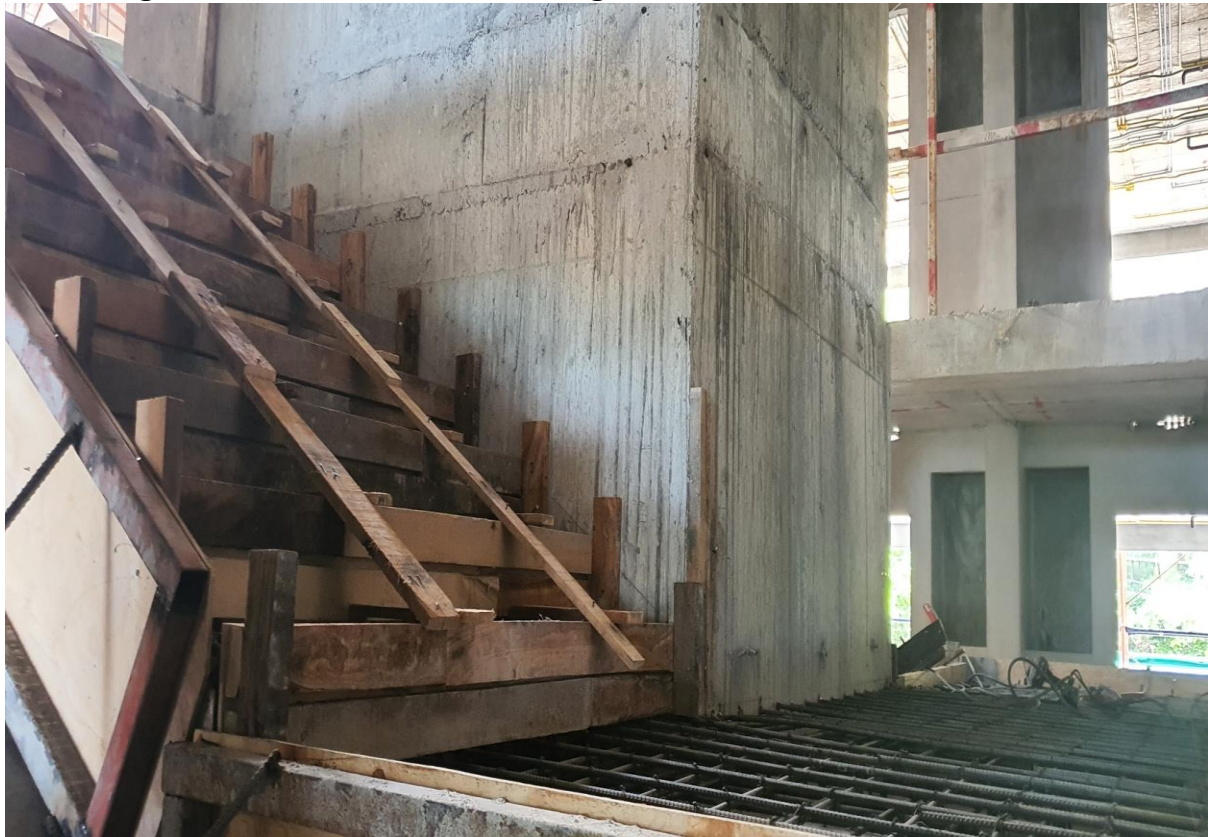
Main Stair Formwork from G floor to 1 st Building 8
