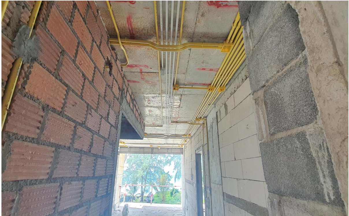
Building 1 st Blockwork, Channel wall conduit work and ceiling conduit work
