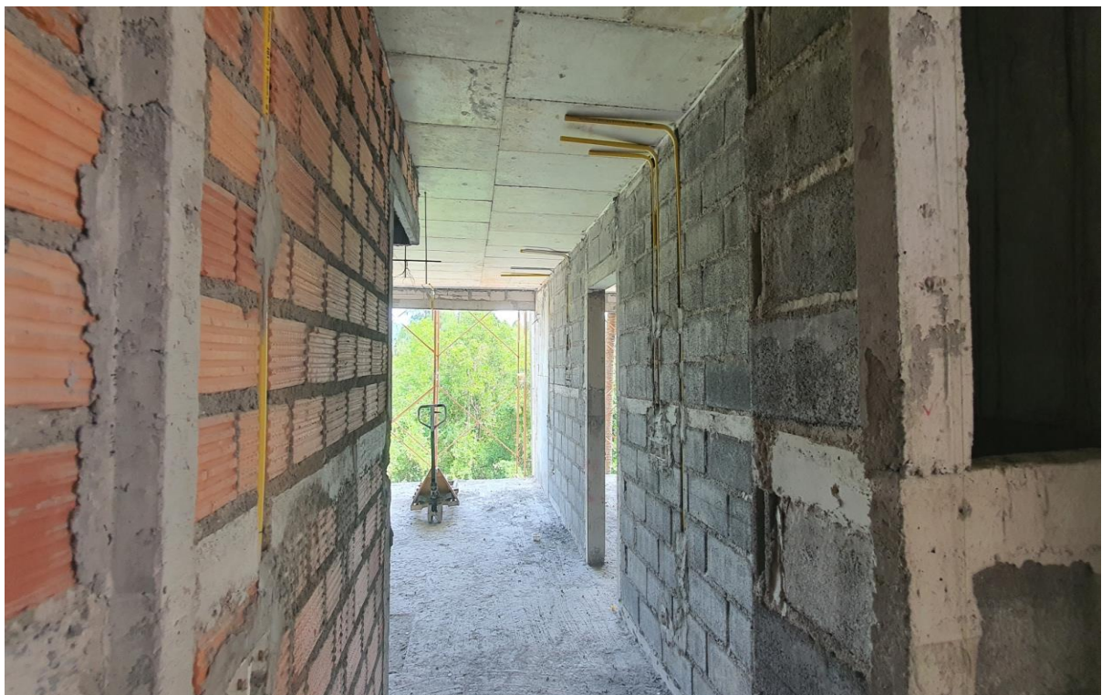
Blockwork and Channel Wall Work 3 rd Floor rear facing units Building 2
