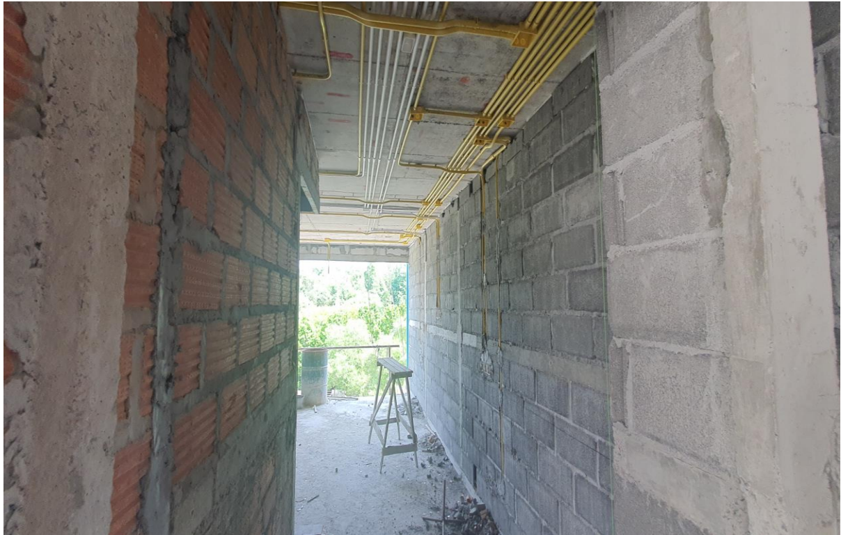
Blockwork and Conduit work 1 st Floor Building 4
