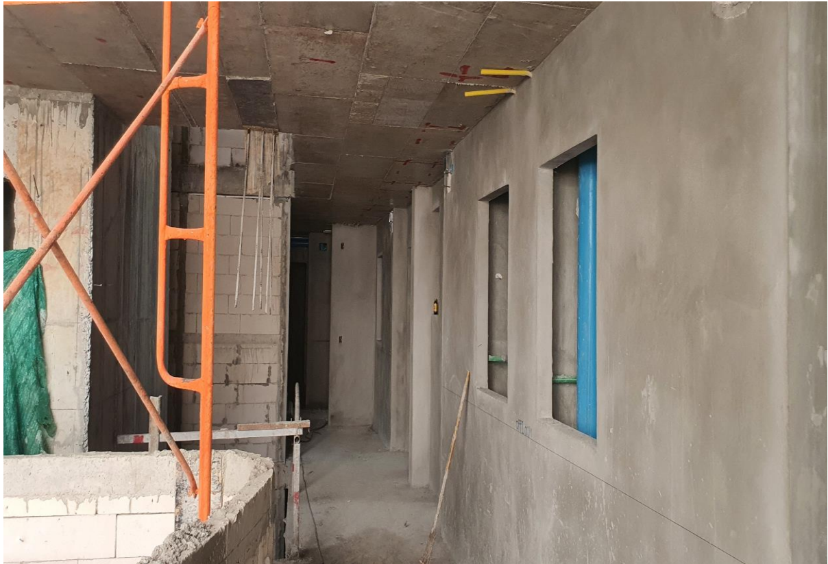
Plastering 3 rd Floor Building 8 corridors
