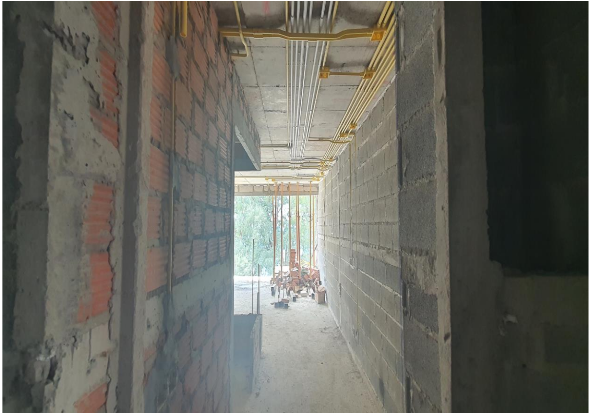
Blockwork and Conduit 2 nd Floor Building 3
