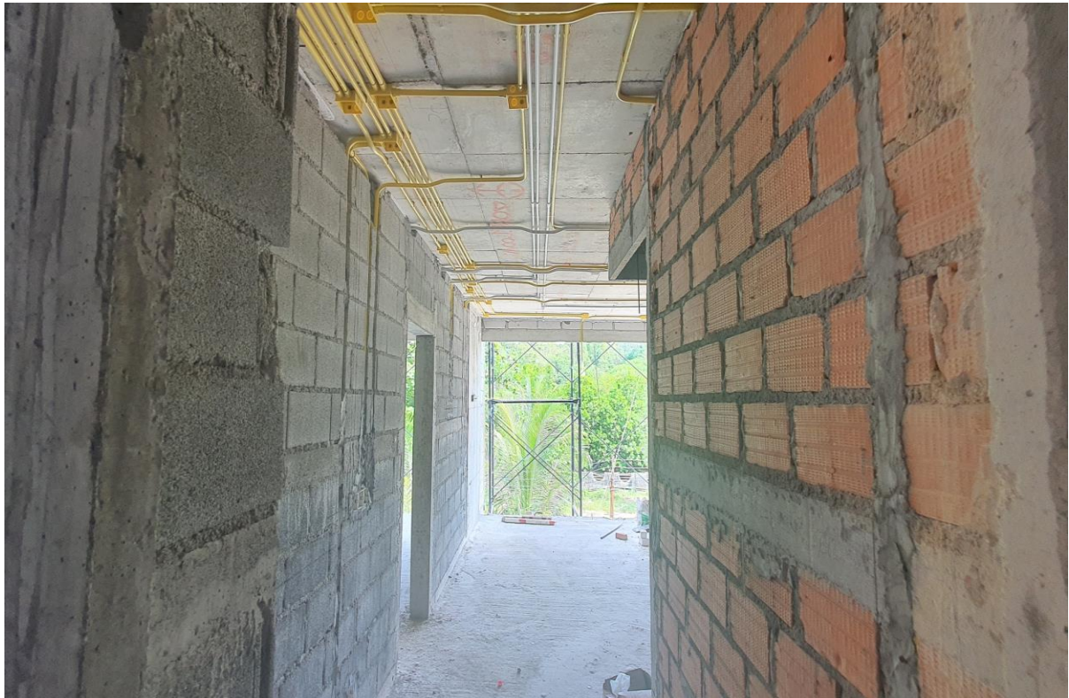
Ground floor building 3 blockwork /Conduit and wall conduit
