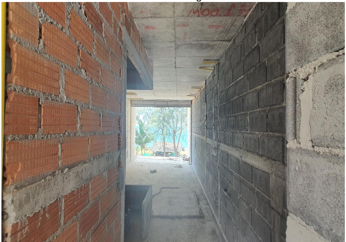
Block work and wall conduit 1 st Floor Building 4
