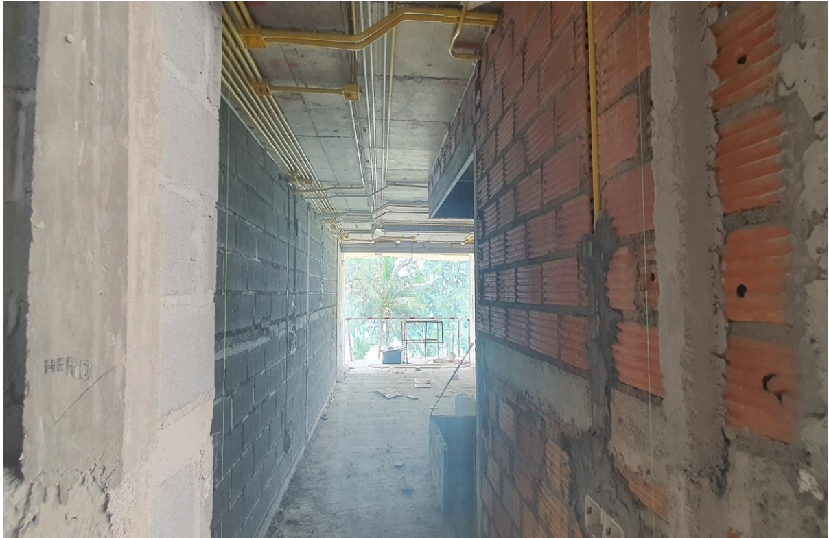
Blockwork and Conduit walls and ceiling 1 st Floor Block 3
