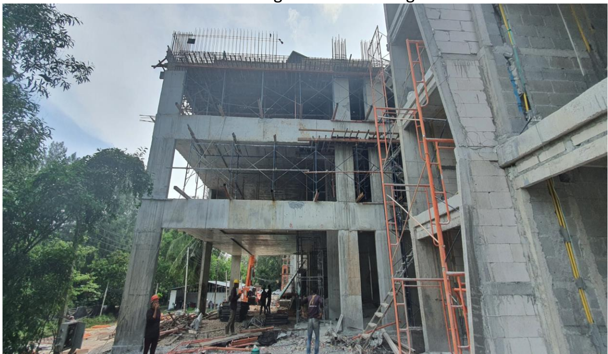
Outside back of Unit 4007 looking toward under Port Cochere Drop off Lobby , formwork of roof slab underway (where the roof top bar will be – can see the areas that will form meeting room and Spa as well above Port Cochere
