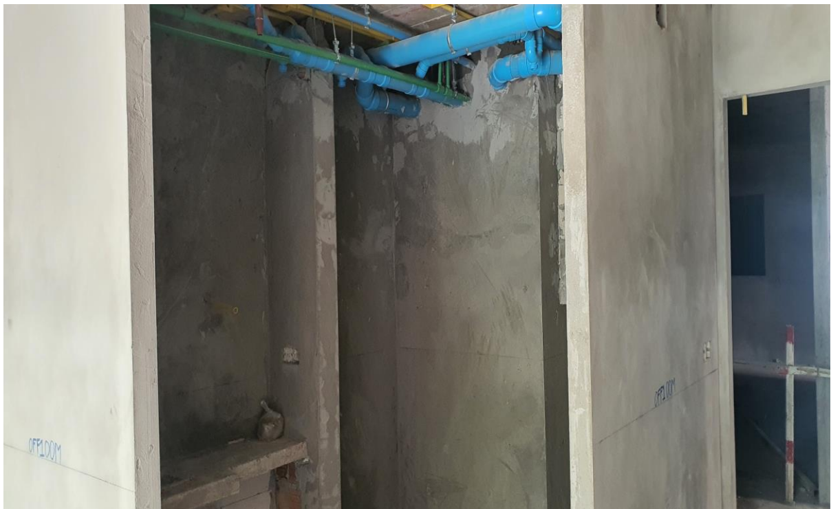
Plastering inside Toilet area 1 st Floor 8
