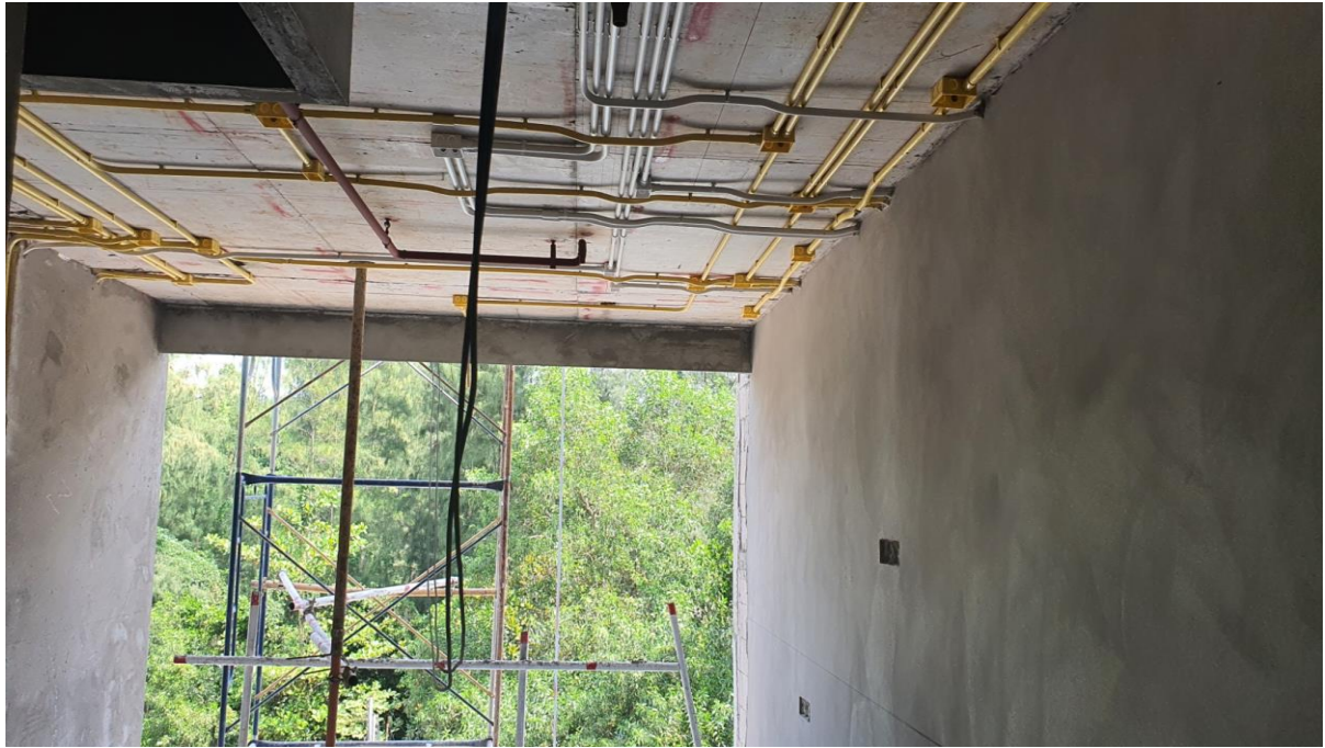
Plastering 3 rd Floor Building 7
