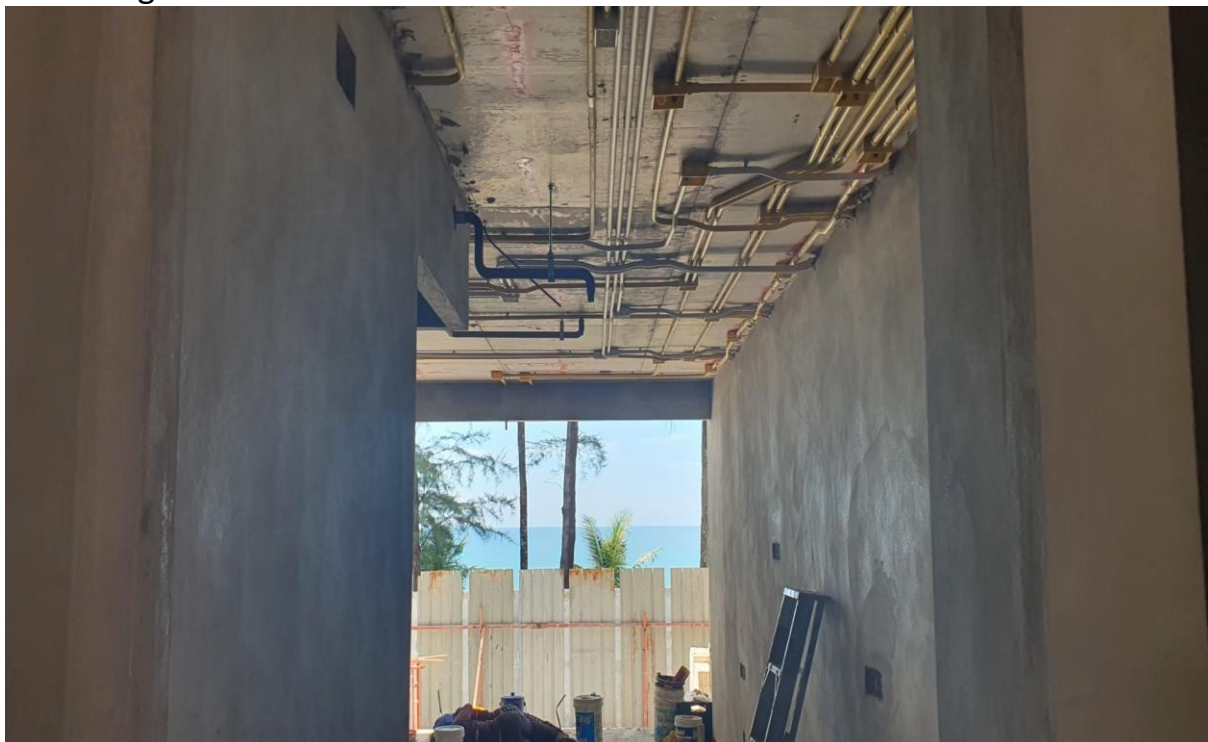
Plaster Inside Room G Floor Building 8
