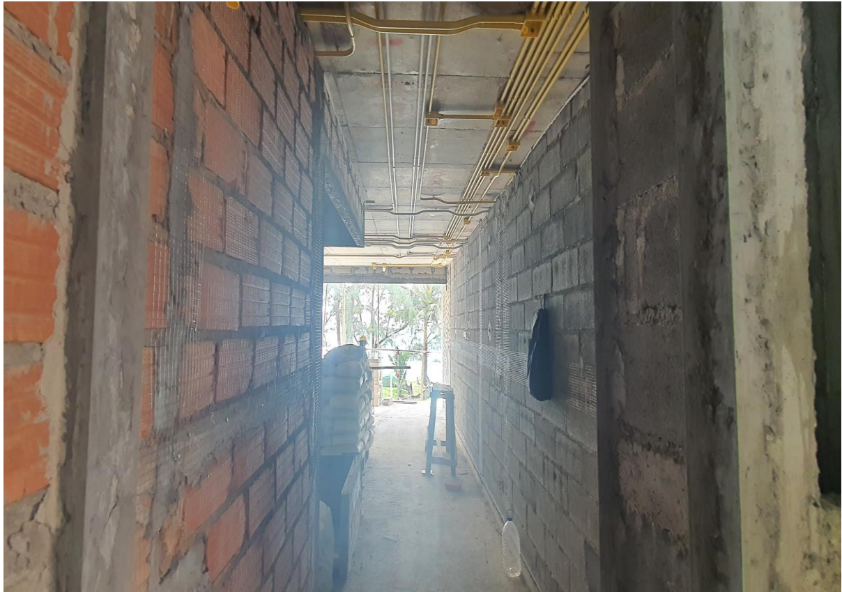
Blockwork /Conduit work inside 1 st Floor Building 4 – prepare netting over conduit /Lintel ready for plastering
