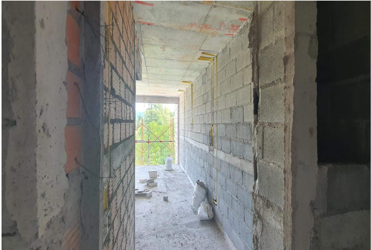
Blockwork and Channel wall conduit work 2 nd Floor Building 2
