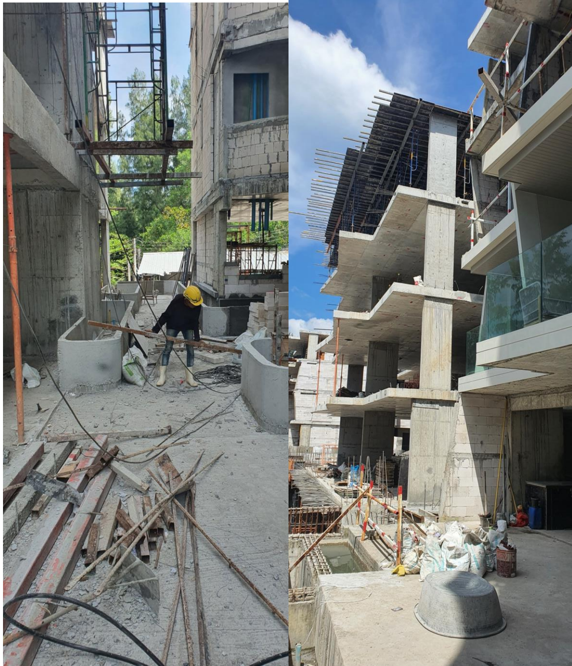
Left Picture is the walkway between 6 & 7 and right picture is Building 6 coming up with the formwork being the roof floor
