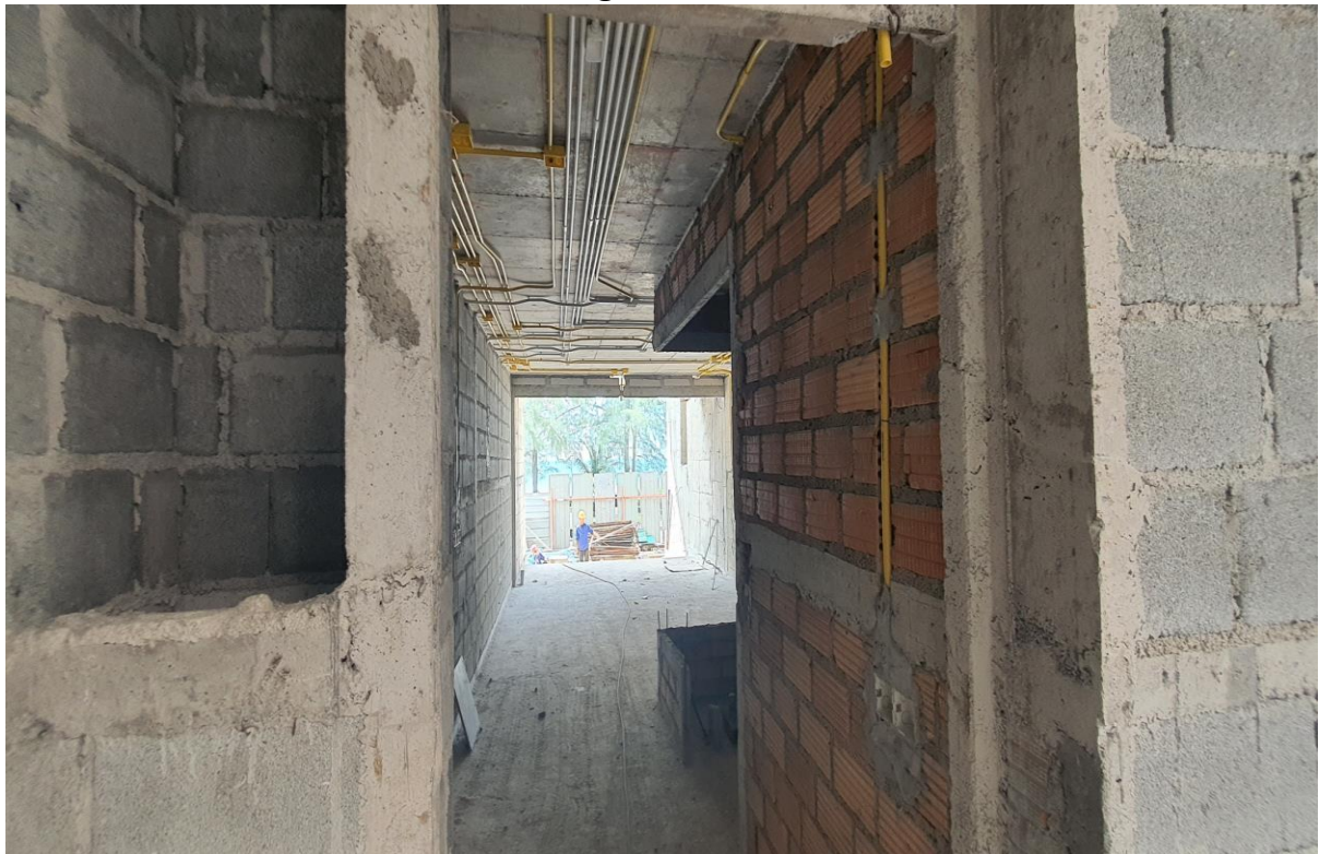
Blockwork Ground Floor Building 3 and channel walls for electrical conduit/back boxes and ceiling conduit work
