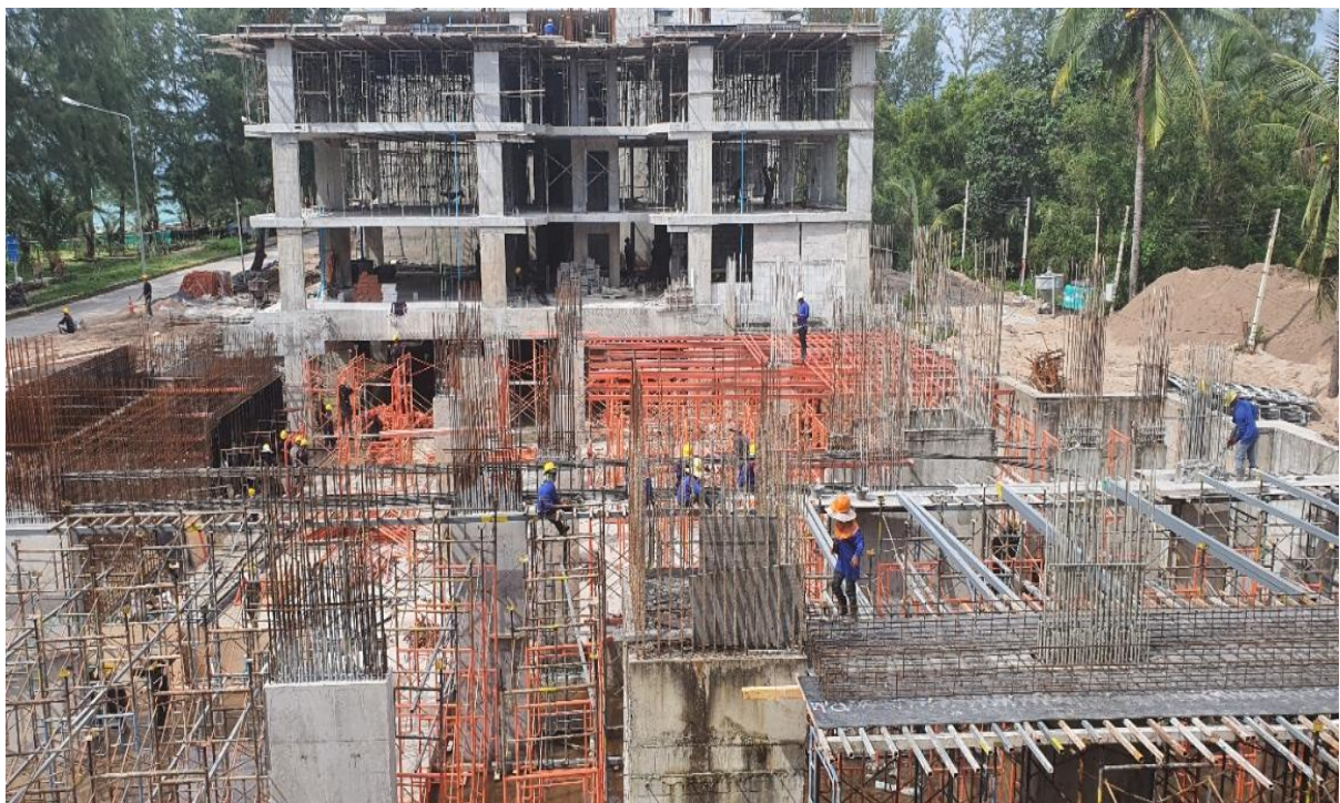
Building 5 & 6 formwork /scaffold ready for G floor
