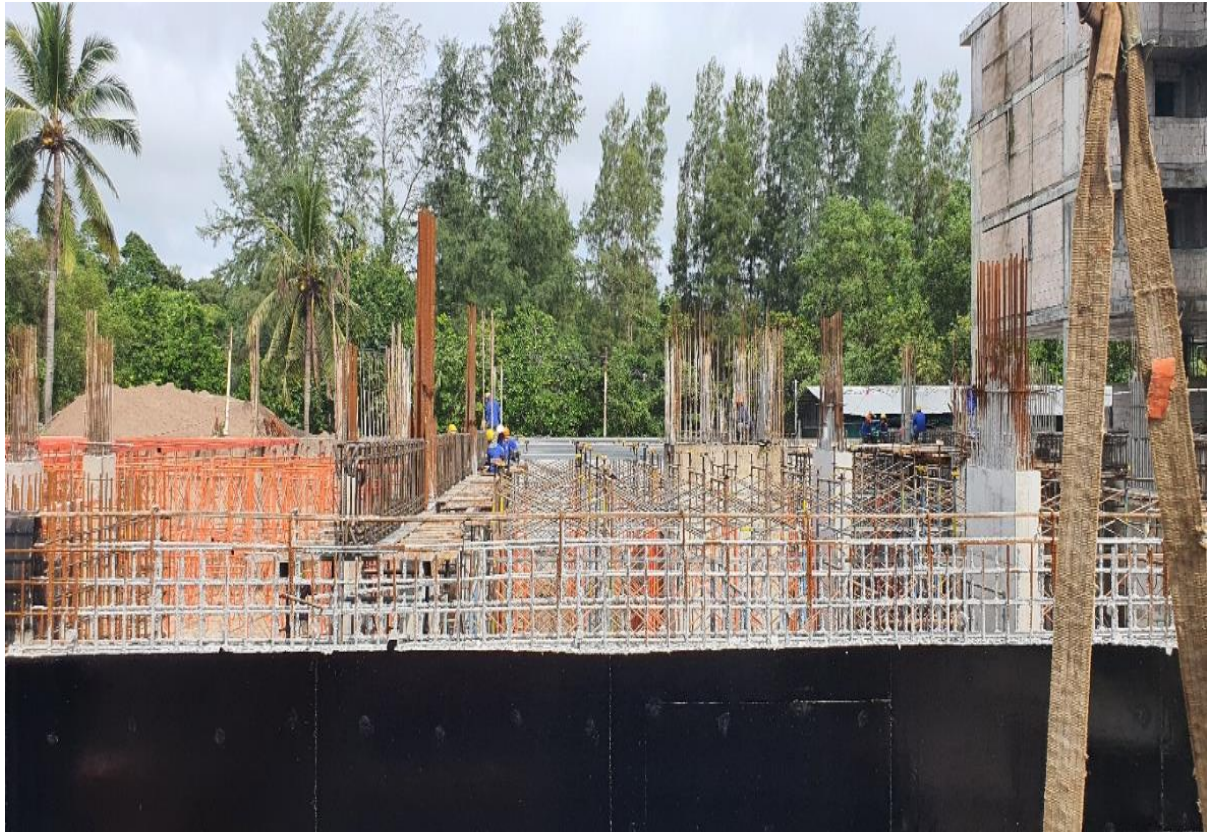
Formwork being done for G Slab building 6
