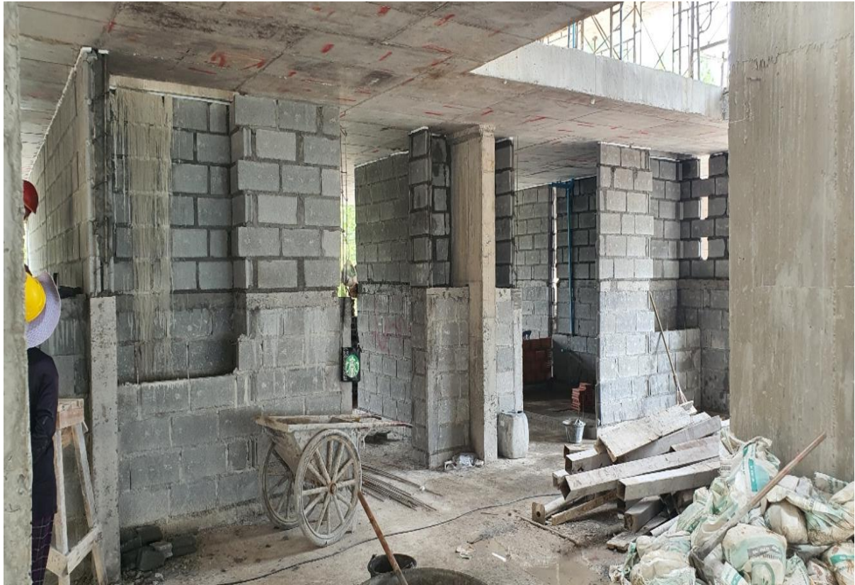
Blockwork Commenced in G floor Building 4 rooms 4006&7
