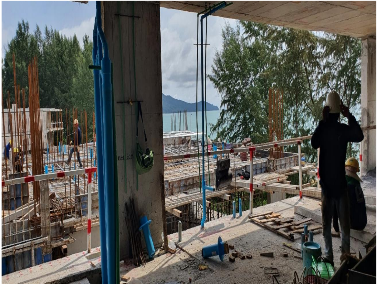
Building 3 looking into 4 at level 3 prepare the slab steel and Post tension sling
