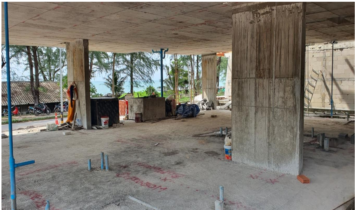
Marking out blockwork G floor Building 4
