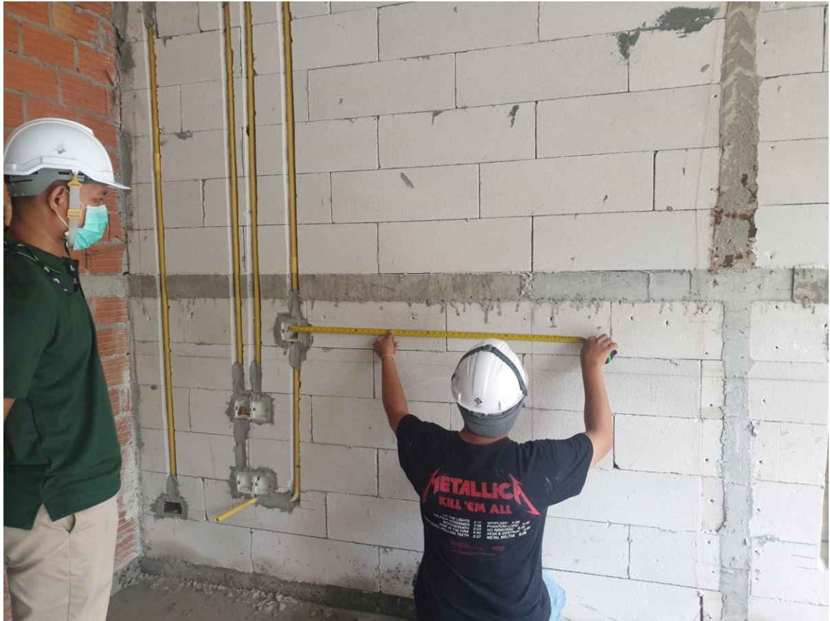
Check/verify levels conduit in walls for switch & Plug
