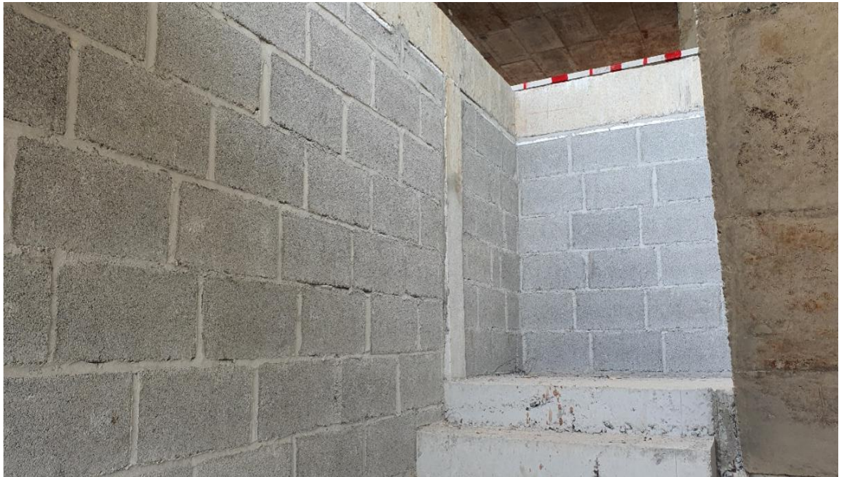
Fire stair Blockwork Building 3 Level 1-2
