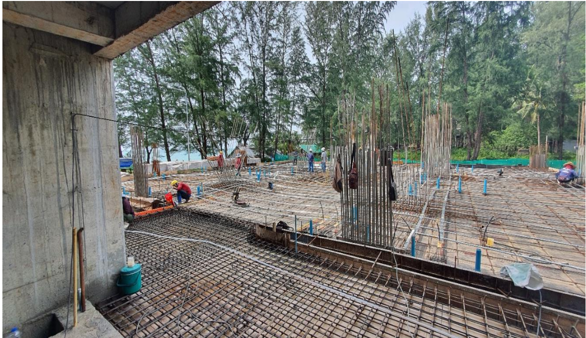
Rear of building 2 overlook Building 1 prepare for pour G Floor slab
