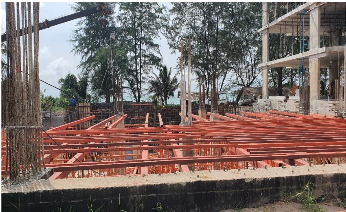
Formwork G level Building 5 – the Lobby /Reception
