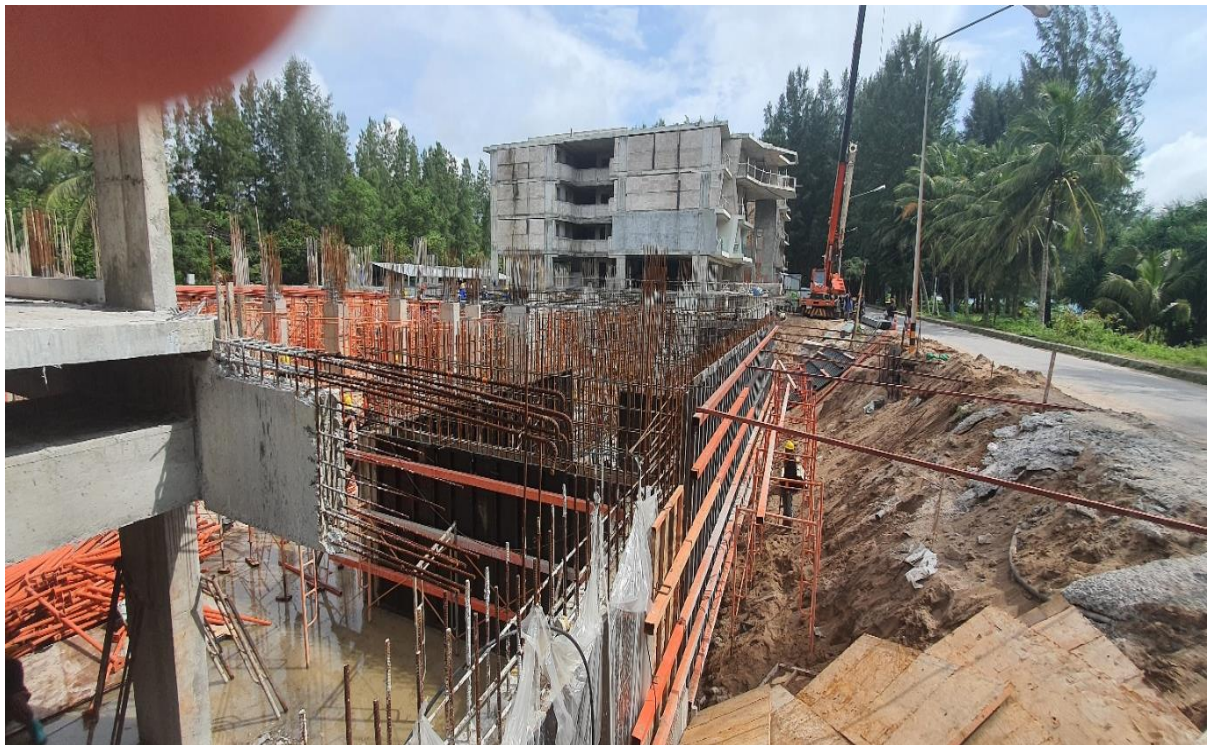
Prepare structure of Pump room/Surge tank
