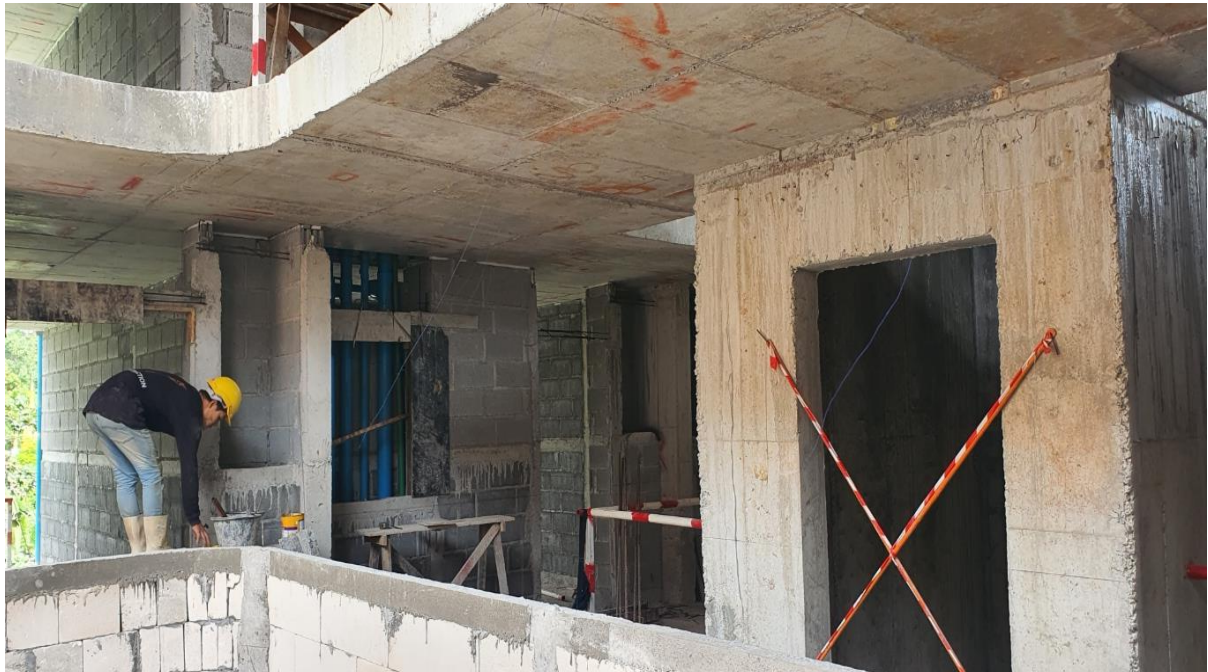
Building 3 Level 2 blockwork
