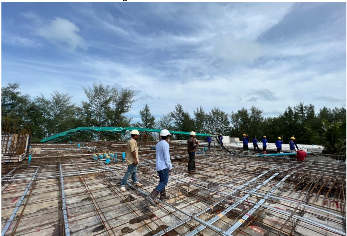
Sleeve work for Slab Building 3 Roof level
