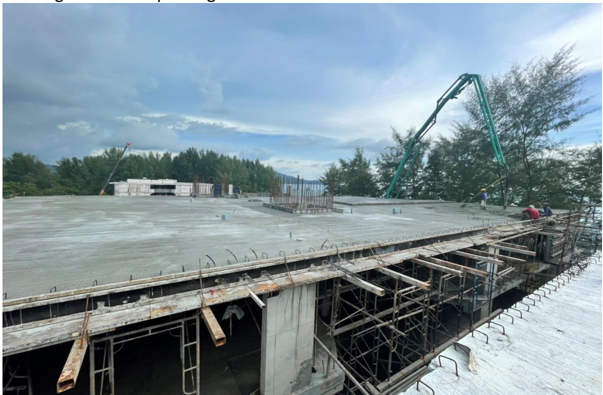
Building 3 Roof Slab pouring
