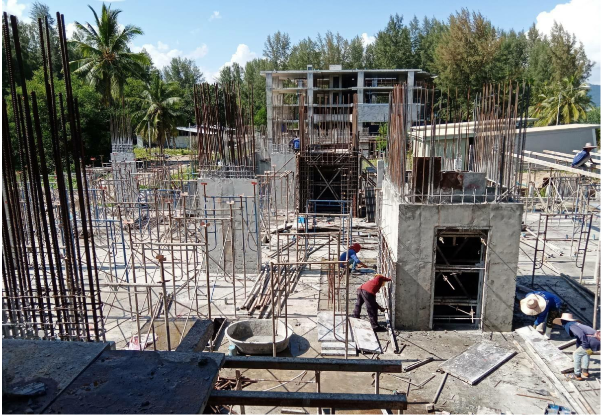
Set scaffold for formwork Slab 3-1
