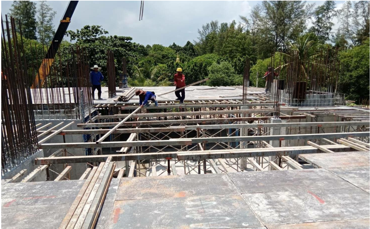
Create formwork Slab 3 -1
