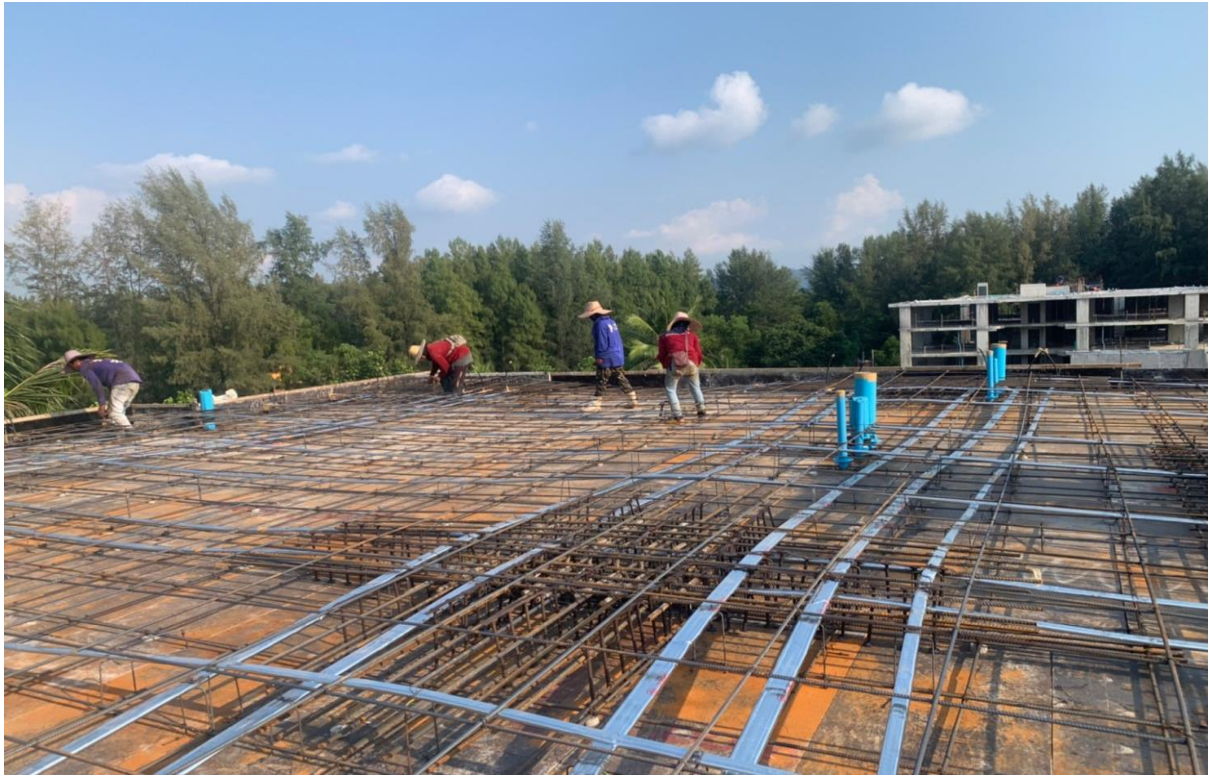
Install Sleeve/Steel/Post tension Sling Roof Floor Building 2
