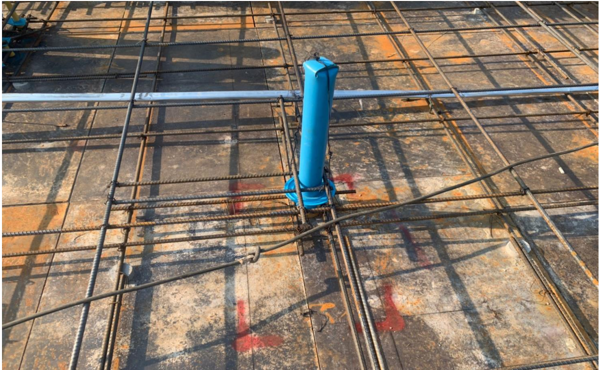
Sleeve through slab for sanitary system Roof Building 2
