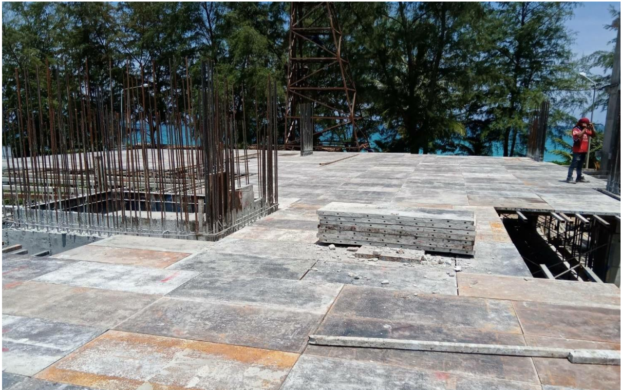
Set scaffold for formwork Slab 3-1
