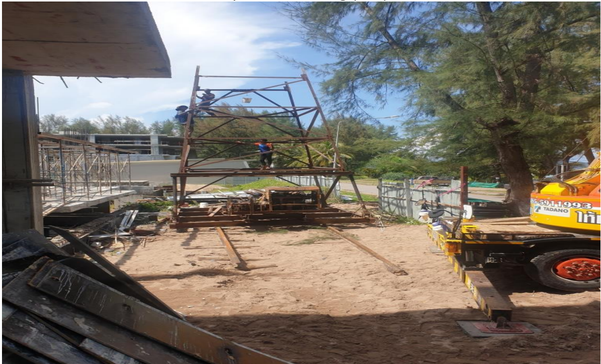
assembly piling machine in pool area in front building 3
