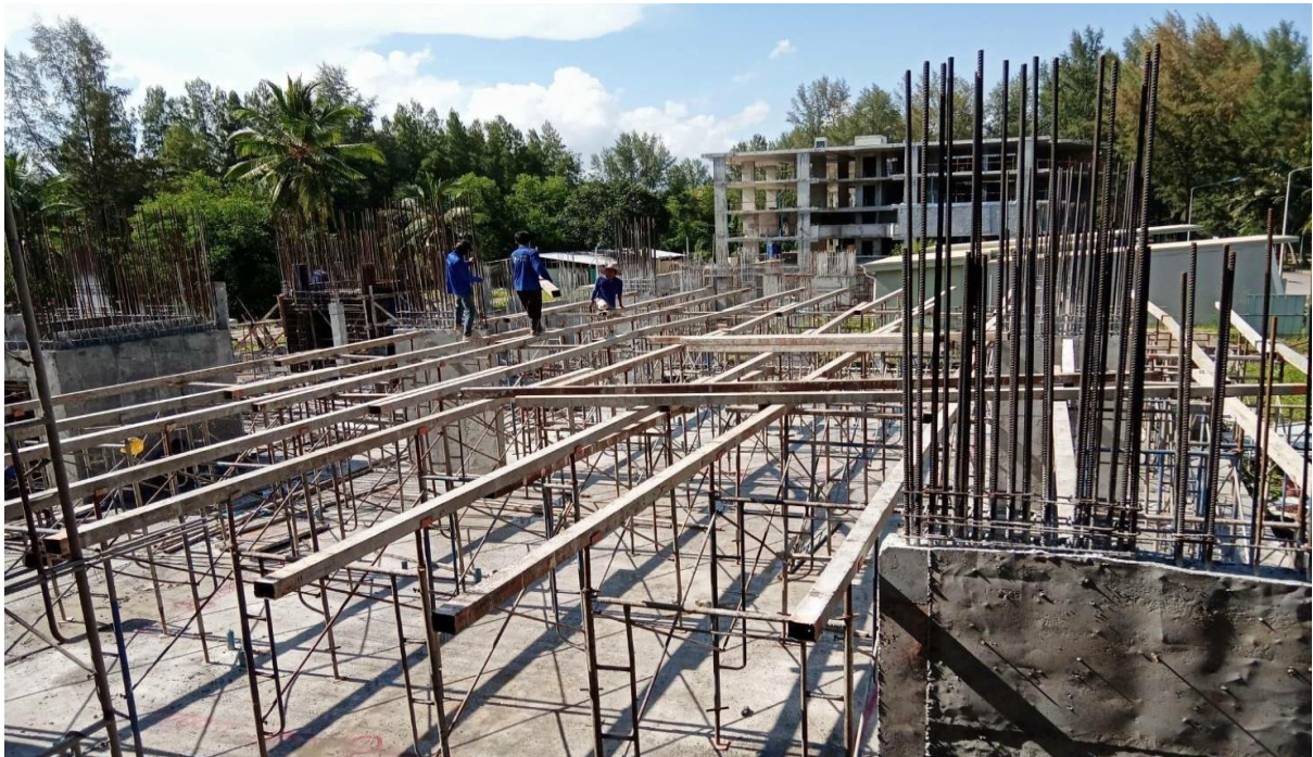
Create formwork Slab 3 -1
