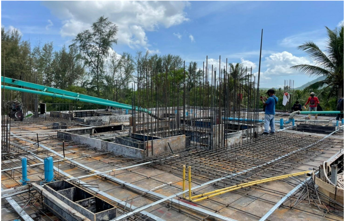
Rebar /Post tension Sling on Slab 2-3 and concrete pump beginning pour of slab
