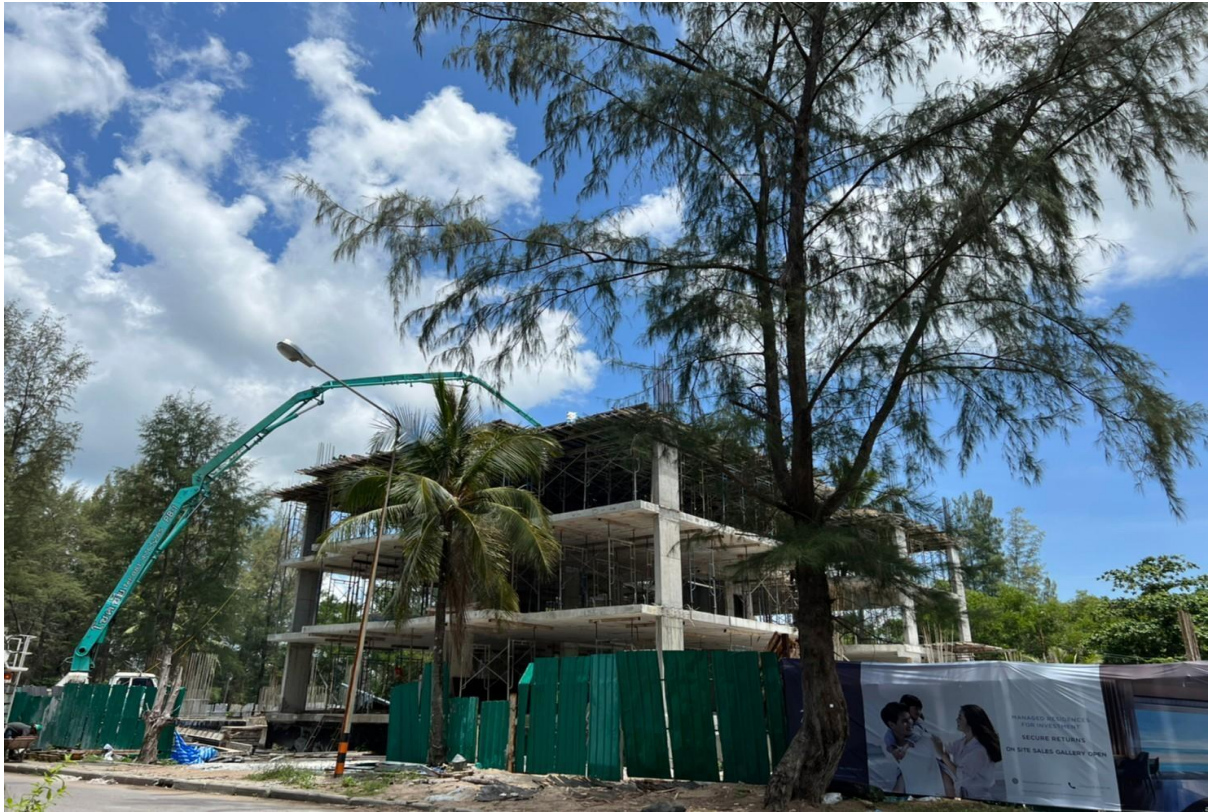
Pouring Slab Building 2 3 rd Floor
