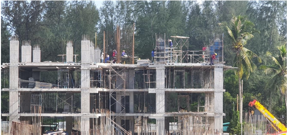
Columns from Level 3 to roof Building 2 and Lift core steelwork
