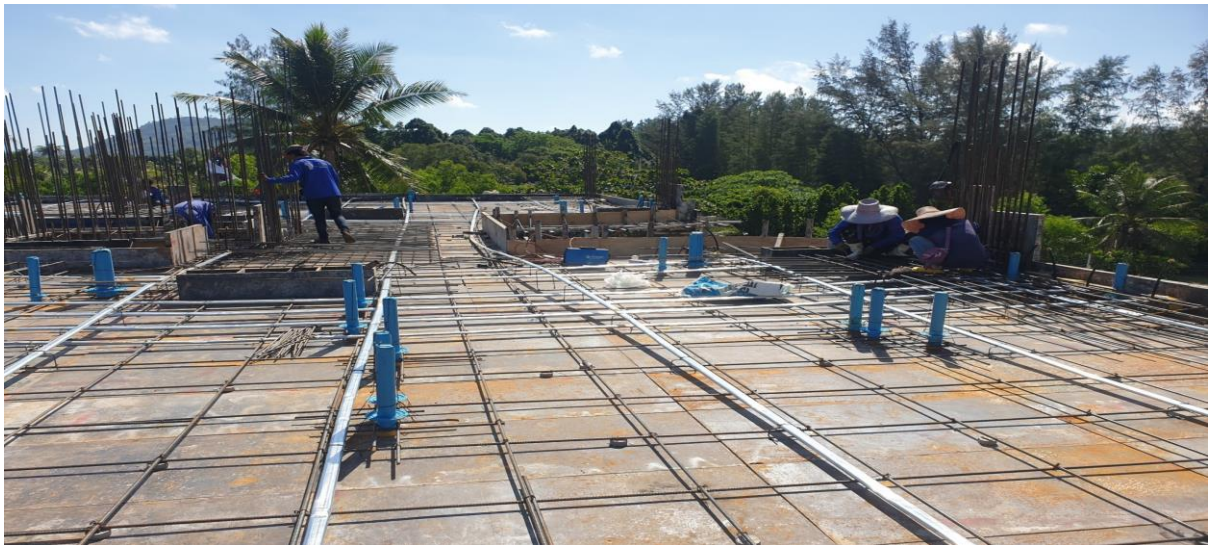
Installing Rebar/Post tension Sling and Service sleeves pre pour Building 2 level 3
