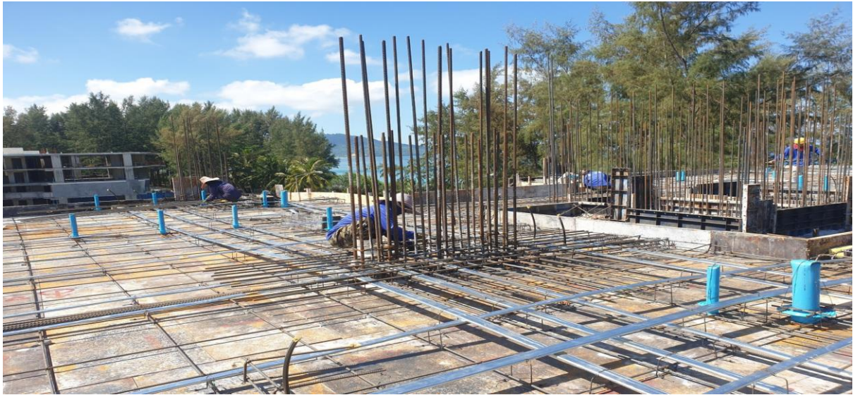
Installing Rebar/Post tension Sling and Service sleeves pre pour Building 2 level 3
