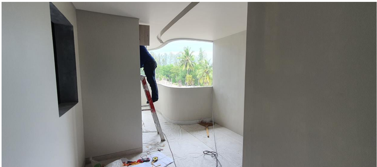
Corridor from 7102 to 7101 – the wall to right hand side does not exist in actual this is just temporary protect top main stair and lift shaft- the curve balustrade wall is part of the finish. The aperture on left is wet shaft of 7102 that will have shaft door fitted
