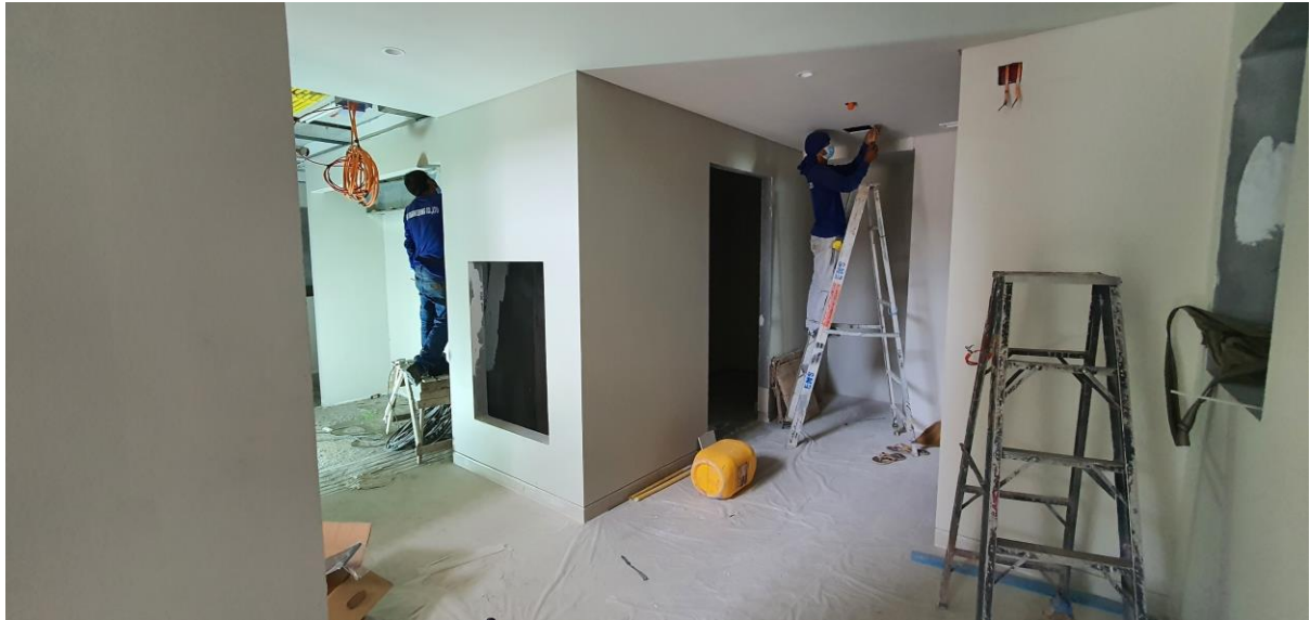
Corridor area – Rh side is wet shaft 7103 – behind ladder centre of pic is service lift (boarded temporarily) the door left of ladder in centre is entrance to maid pantry, left of maid pantry the square hole is Fire Hose cabinet aperture, left side ladder is EE cupboard for electrical services
