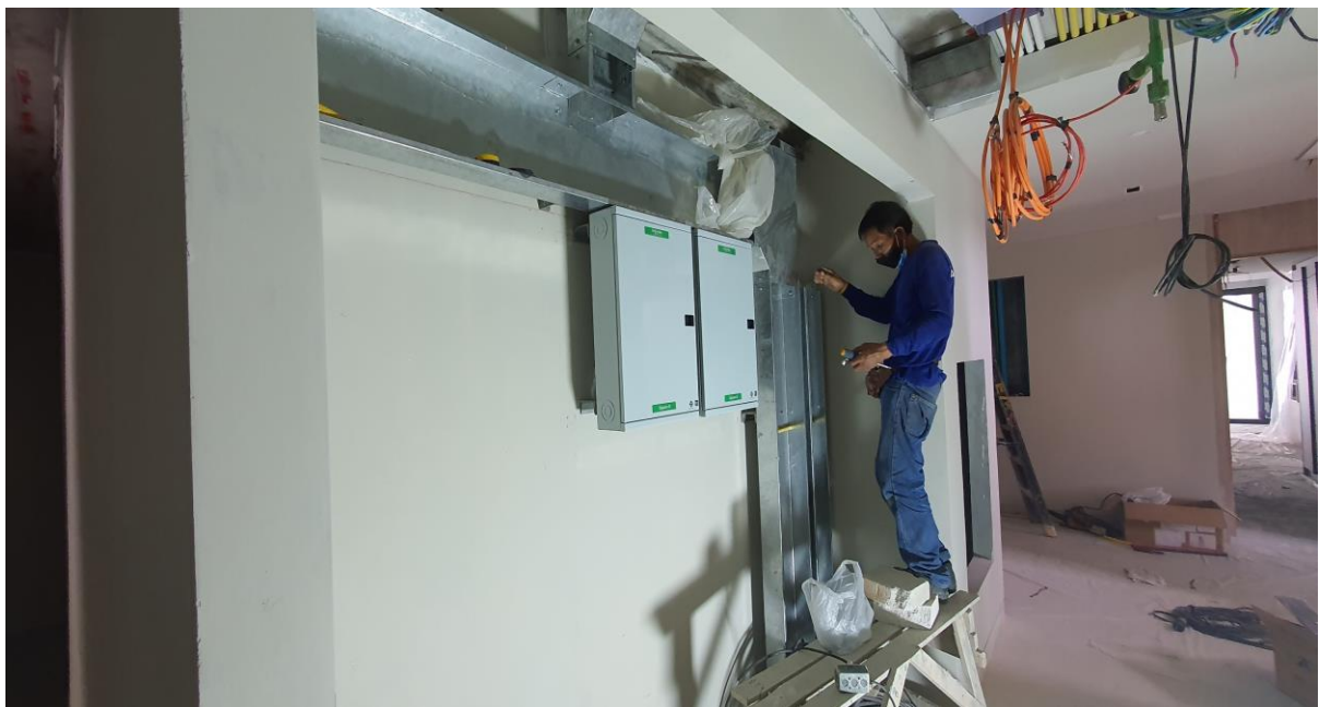
Wideway installation in EE cupboard and DB power box installation for power 1 st floor building 7, sub distribution boxes and sub breakers are contained in the electrical shaft for each room
