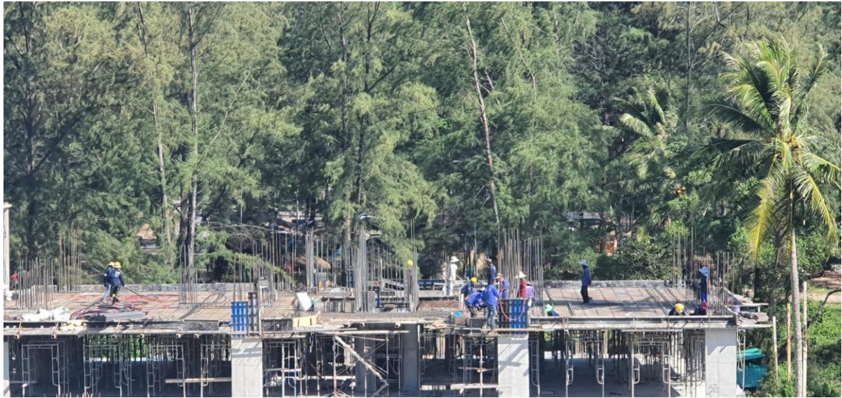
Formwork Building 2 Slab 2 Install bottom steel and start Post tension Sling
