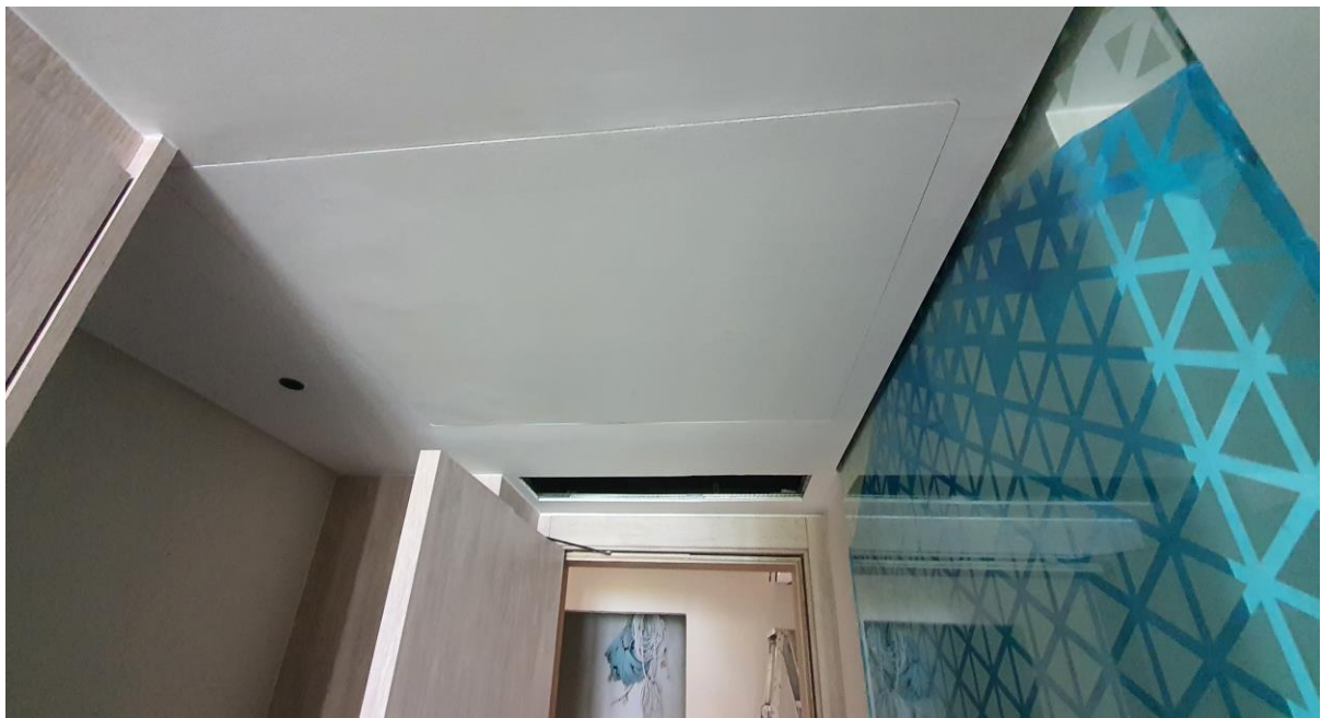
Revised Air Con hatch with magnetic locking (from Show Mock to actual)
