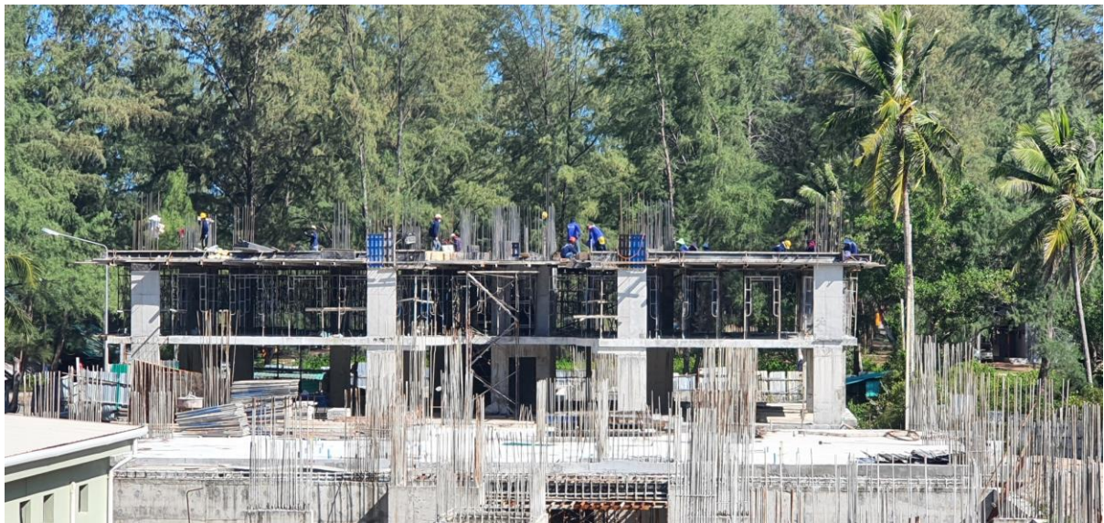
Formwork Building 2 Slab 2 Install bottom steel and start Post tension Sling
