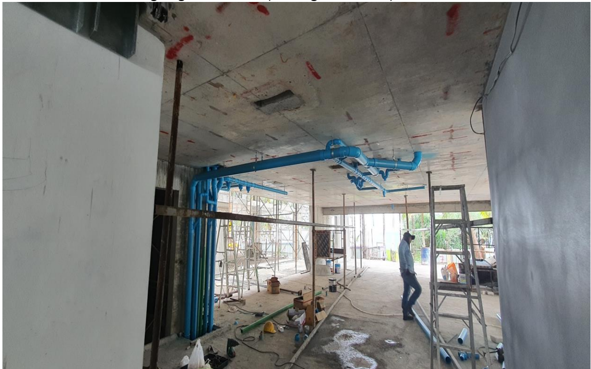
Sanitary sleeve for room 7103 7104 coming down from floor into area ceiling G floor and across to wet riser shafts to exit building
