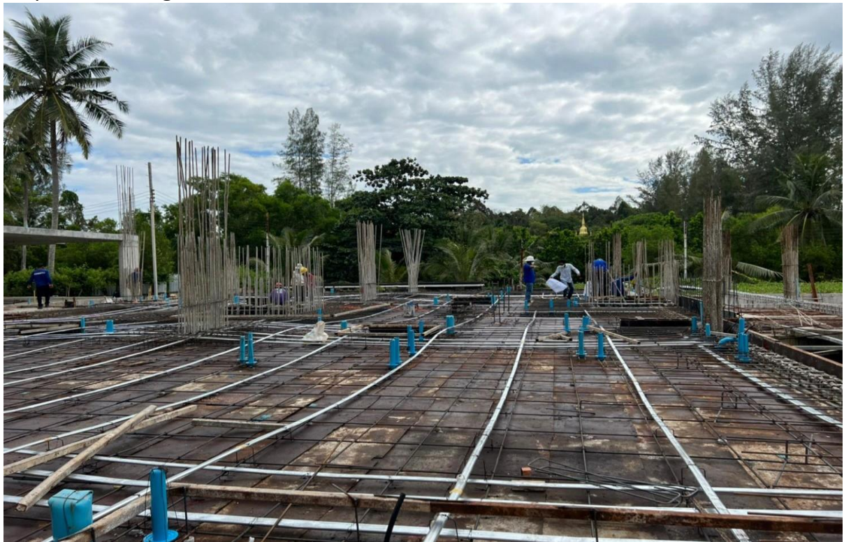
Check Sleeving slab 3G
