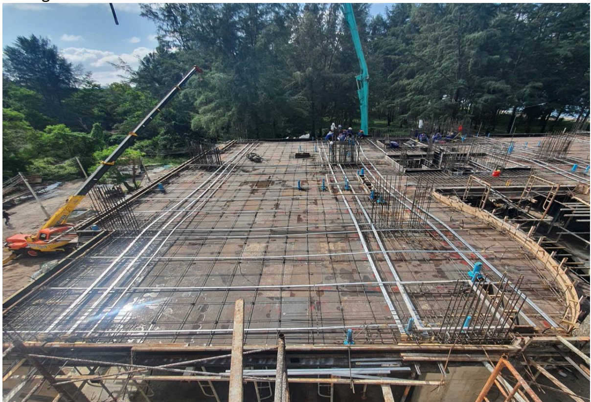
Poring slab & 2 nd floor
