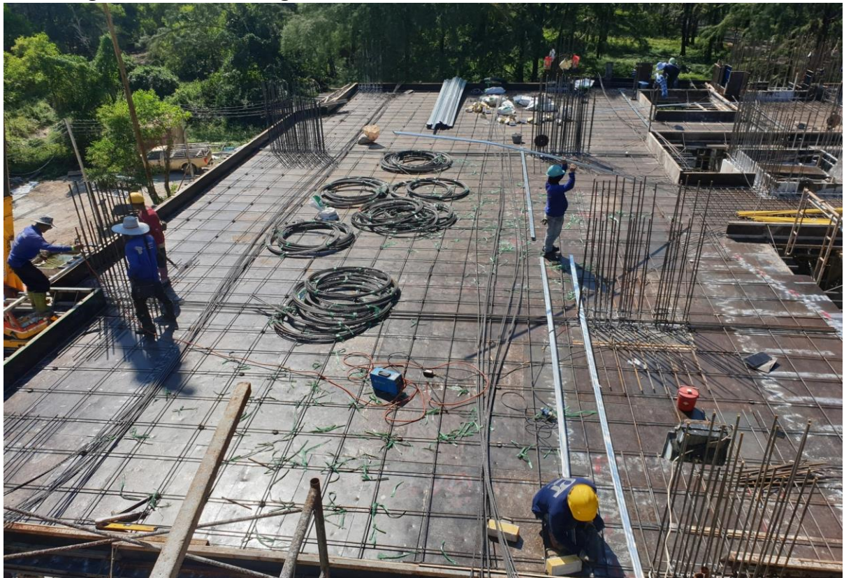
Installing Post tension Sling Slab 8 2 nd floor
