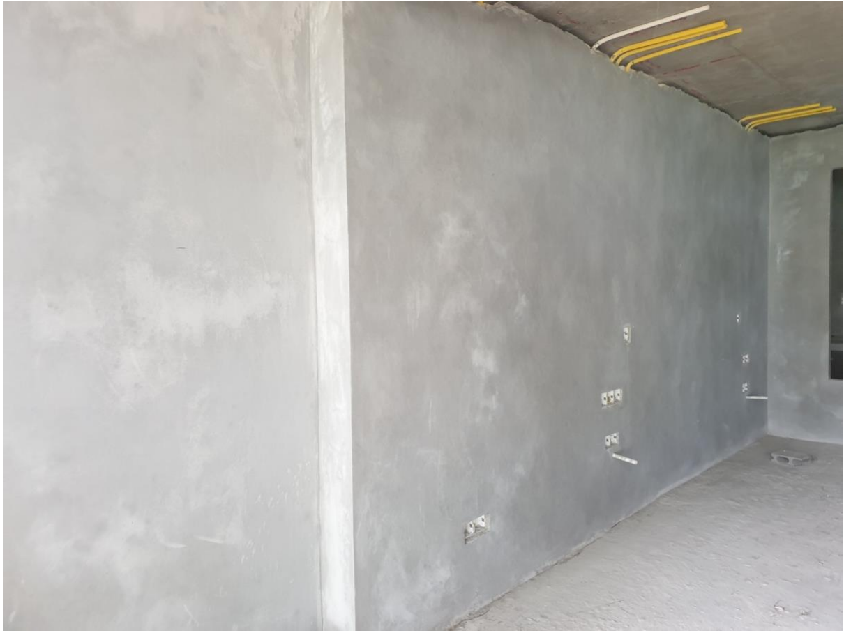
7102 Walls Bedhead with electrical 1 st Fix back boxes
