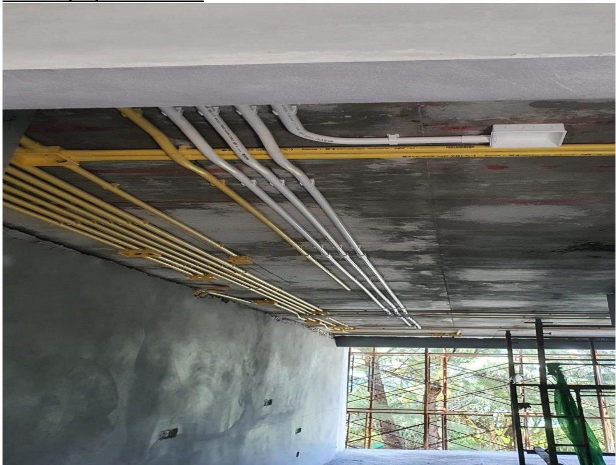
7102 Conduit for Electrical Circuits (Yellow) IT & Communication (White)
