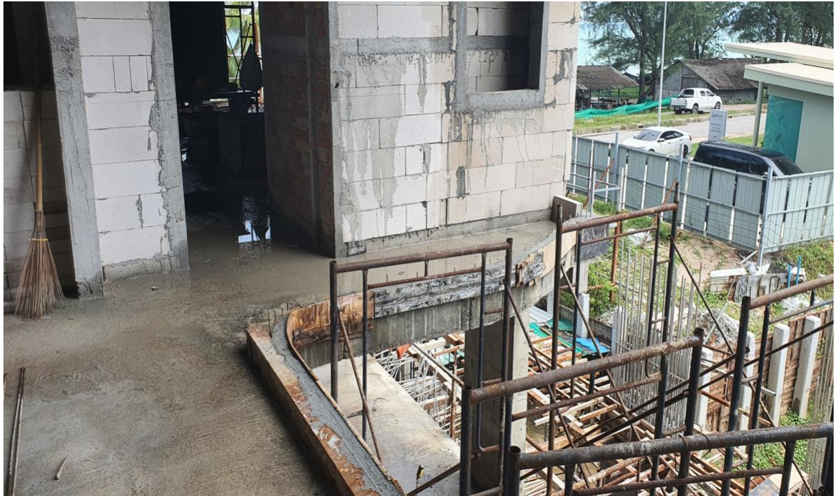
Prepare kerb for Balustrade wall 7-1 in front of 7101
