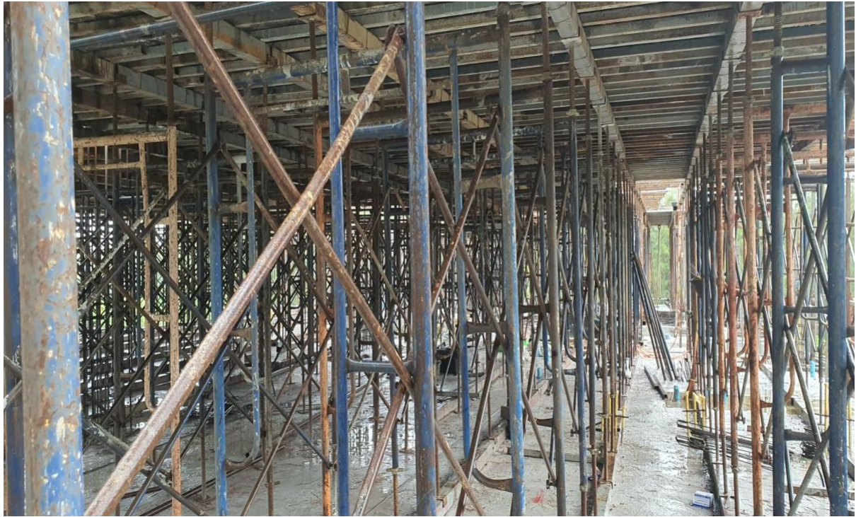
Scaffold support Roof Slab 7
