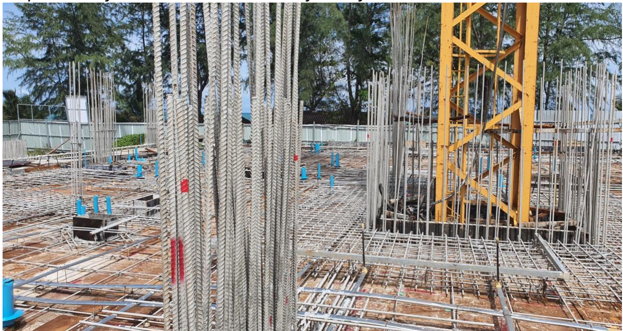
Slab 3-g Formwork/Steel and Post tension sling ready
