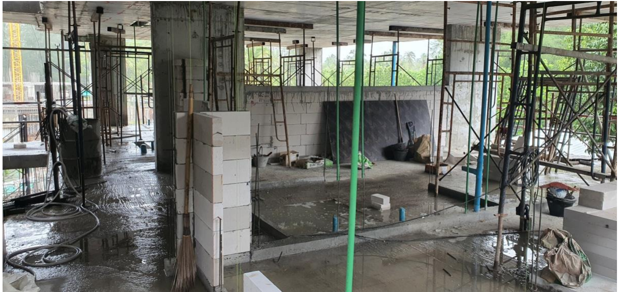
Blockwork commencing garden view room (7105-7108) 1 st floor 7
