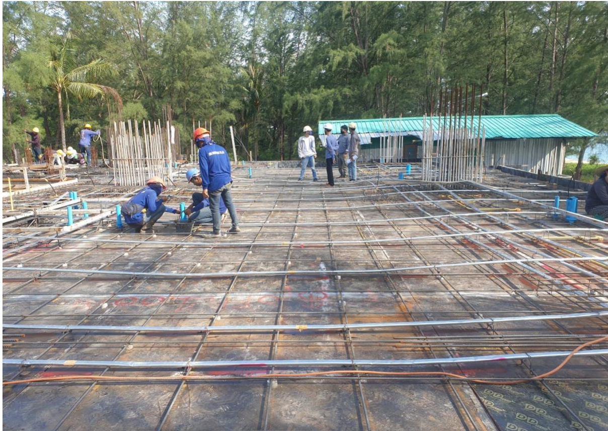
Sleeving preparation Slab building 8- Floor 1
