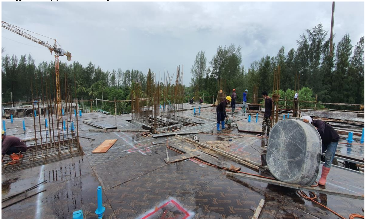
Formwork Building 7 floor 3 – Sleeving installation
