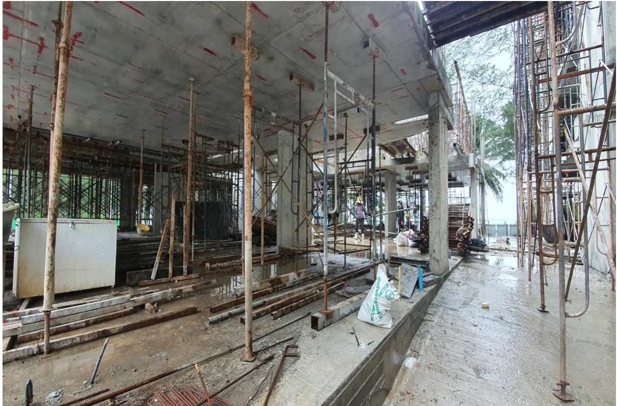
Formwork being removed from underside slab 8-1
