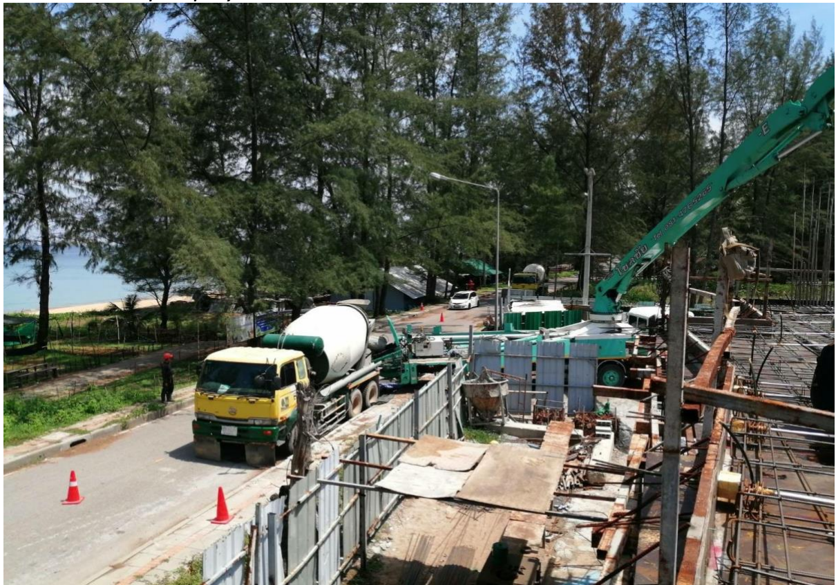
Ready mix arrivals into the concrete pour Building 2 – 1
