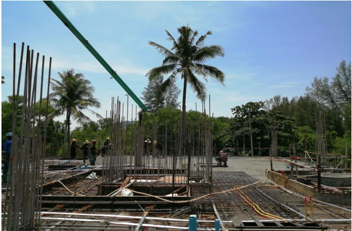
Building 2 Slab 1 pouring guest elevator area in foreground
