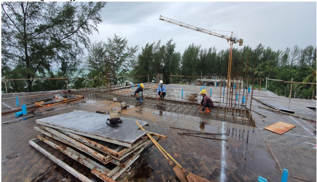
7-3 Formwork and Band Beam steelwork installation (thicker structure area to support Type F Terrace extension)
