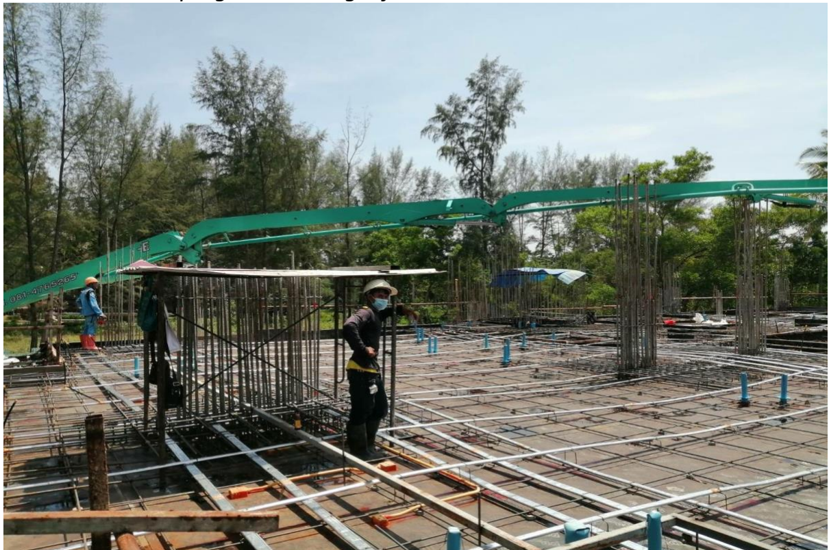
Concrete pump ready for Building 2 floor 1, Post tension cable system visible in the aluminium conduits
