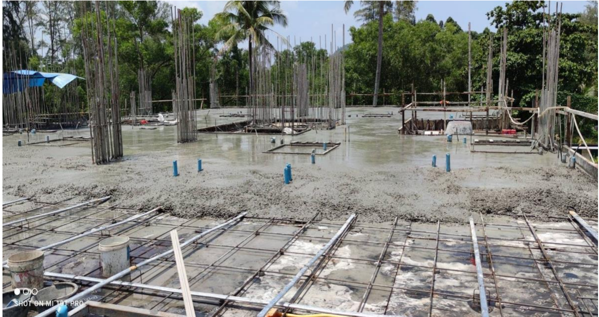
Concrete Pour in progress building 2 floor 1
