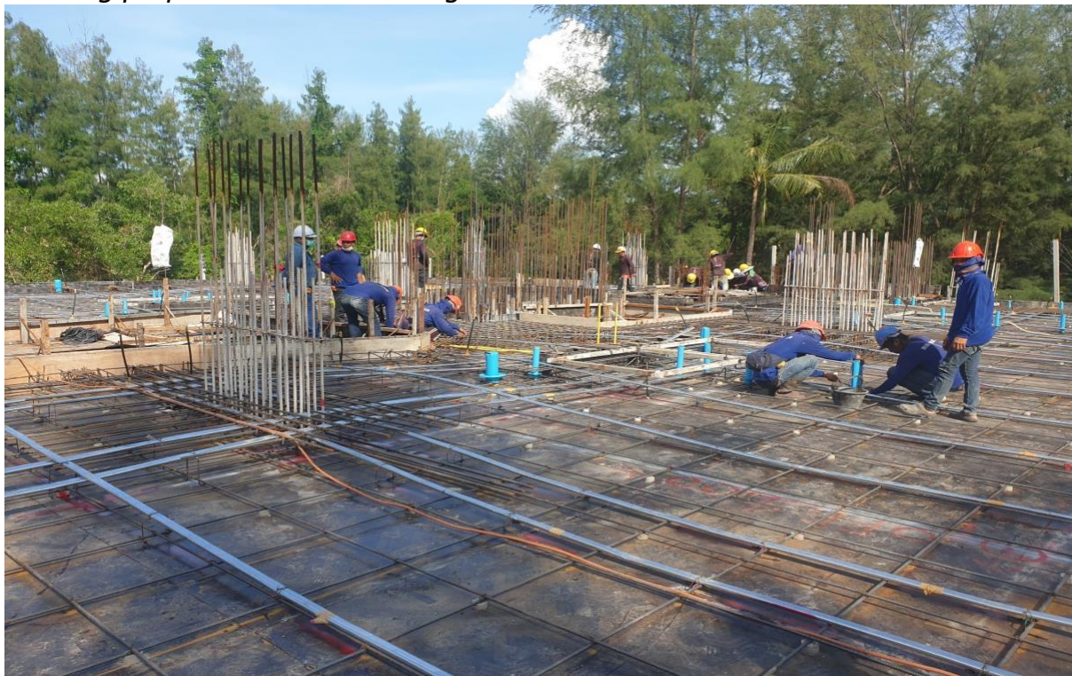
Preparing Post tension sling/Sleeving and top rebar for Slab 8-1
