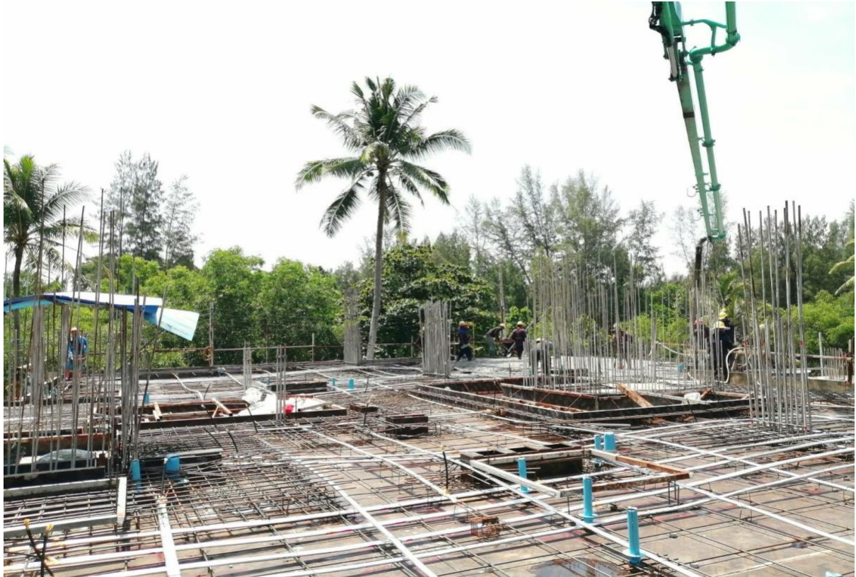
Concrete Pump deployed on Slab 2 -1
