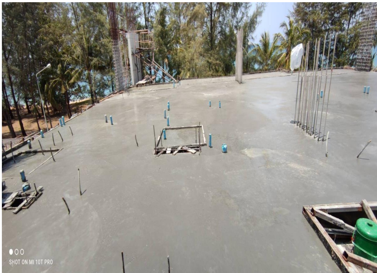
Poring Concrete 7-2
