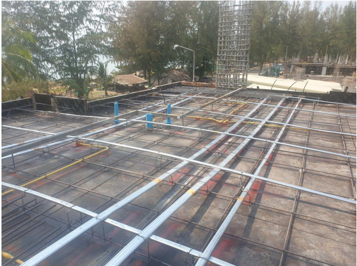
Post tension cabling Slab 7-2
