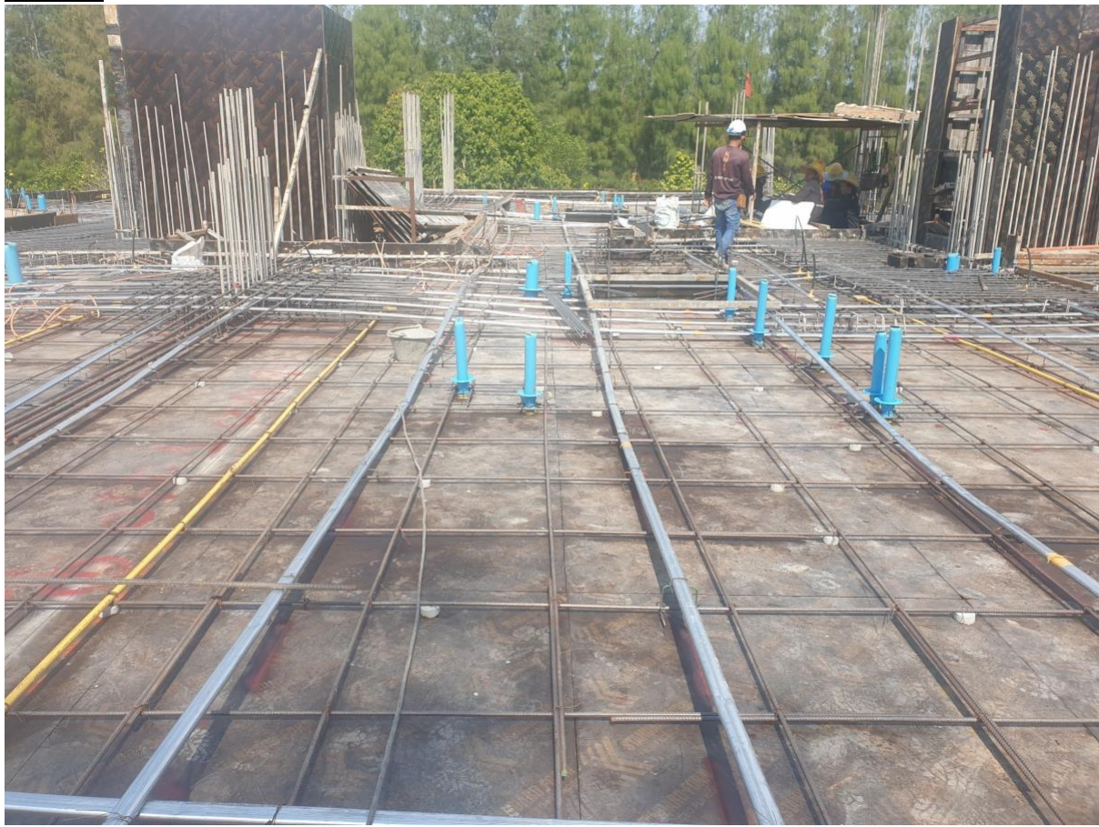
Steelwork and sleeving Slab 2-1
