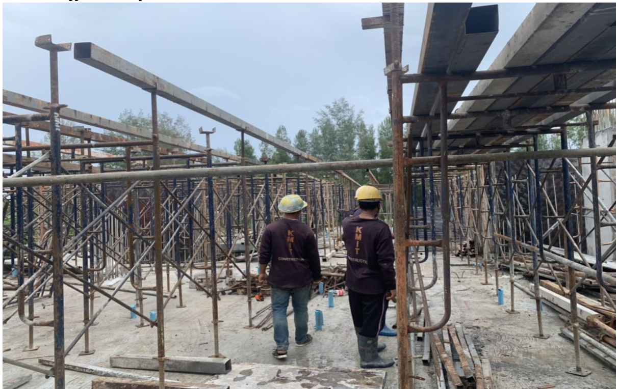
Erect scaffold 7-3 floor
