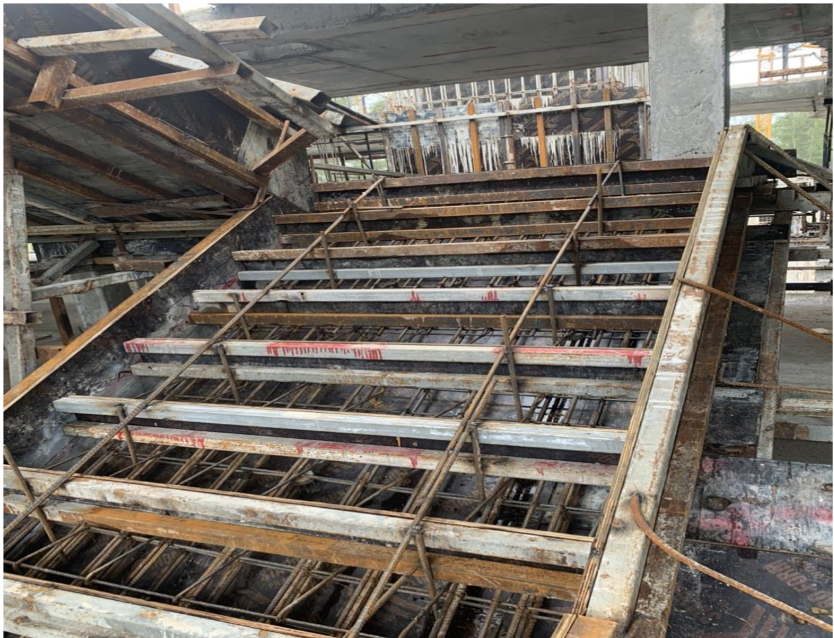
Formwork Fire stair 7-1 to 7-2
