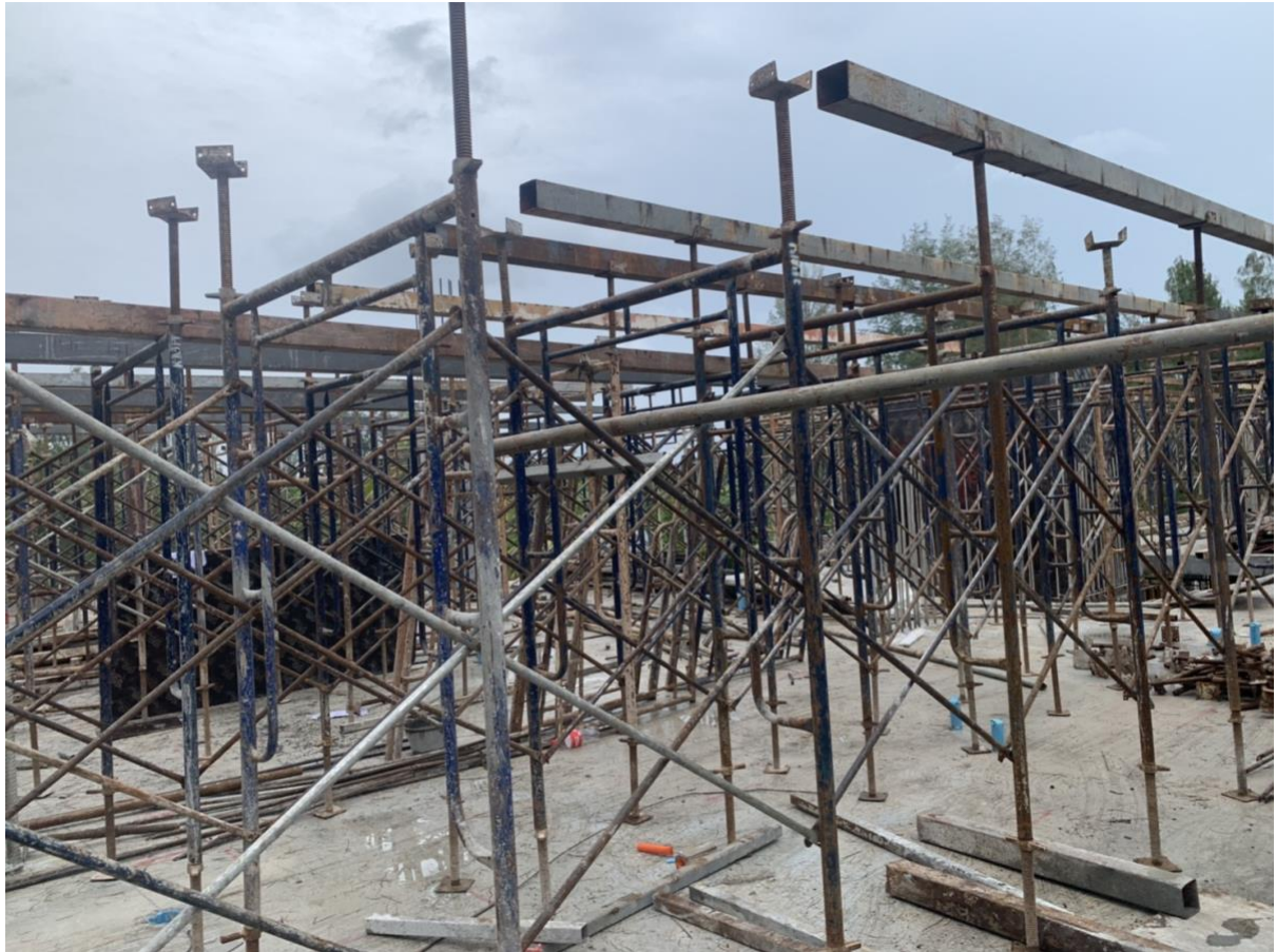
Erect scaffold 7-3 floor
