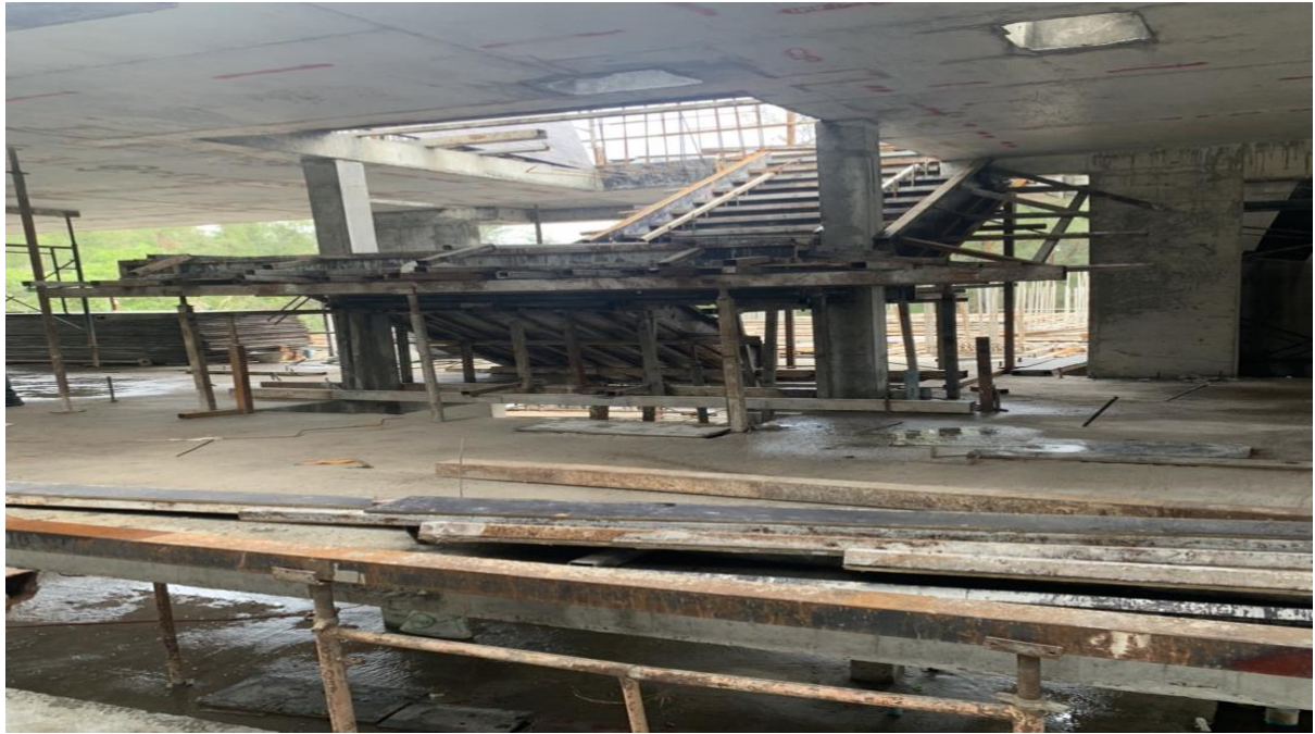
Formwork Fire stair 7-1 to 7-2
