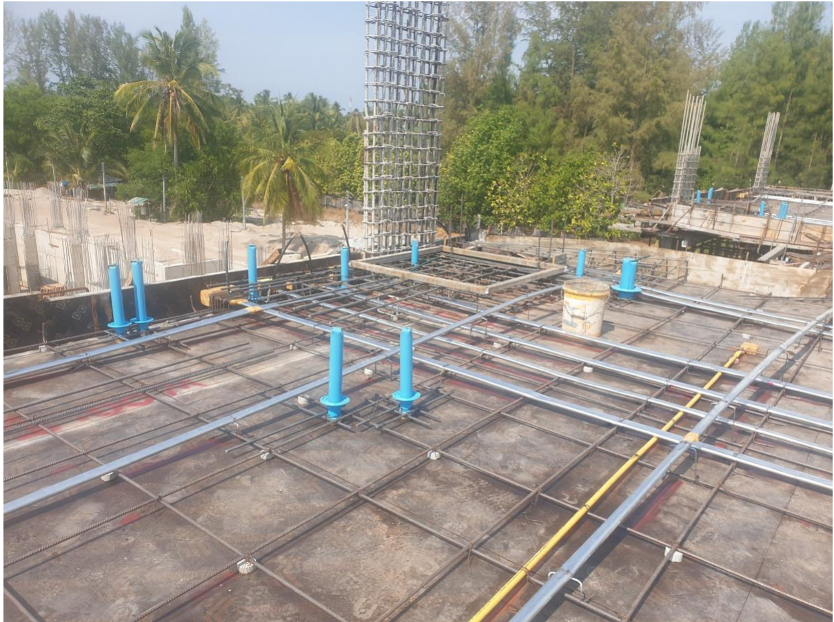
Steelwork and Sleeving 7-2
