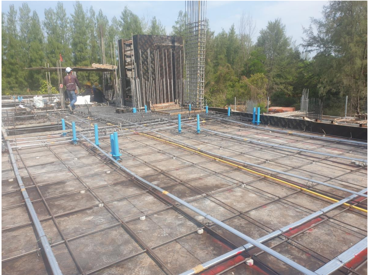
Slab steelwork 7-2
