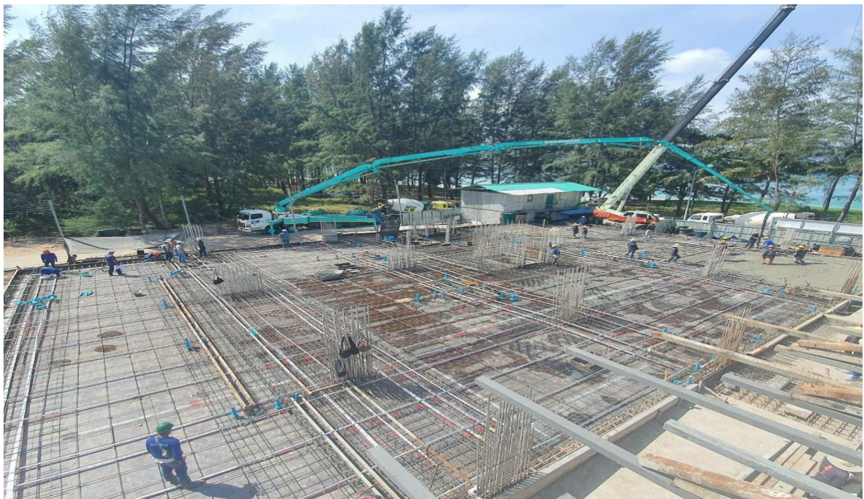
Slab pouring Building 8 G Floor
