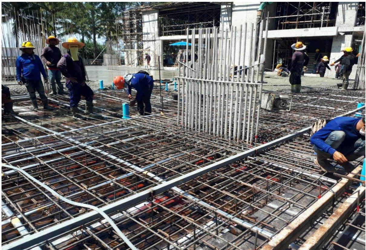
Slab Building 8 on pouring day can see the steelwork and Post tension cabling slings
