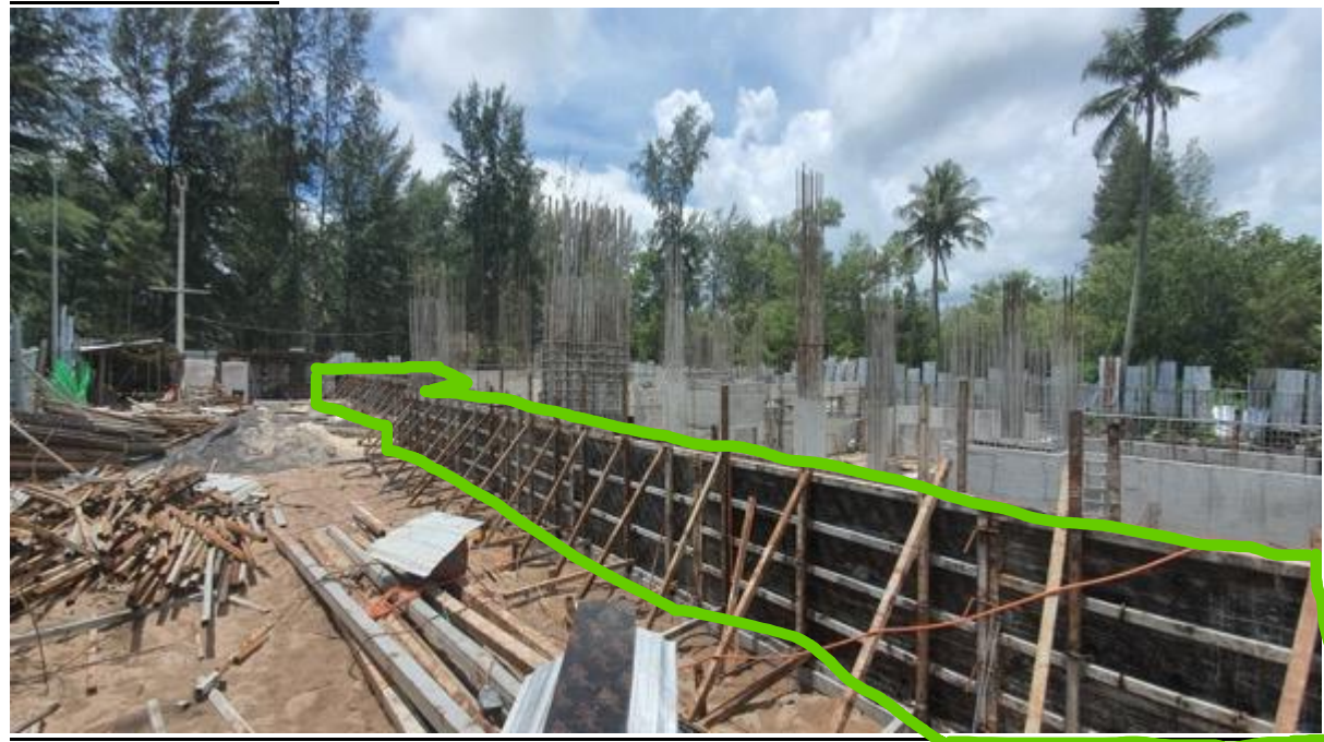
General area building 3 looking towards 2 and 1 – note columns poured to GF level and green cloud area is formwork retaining wall going up from current level to GF level
