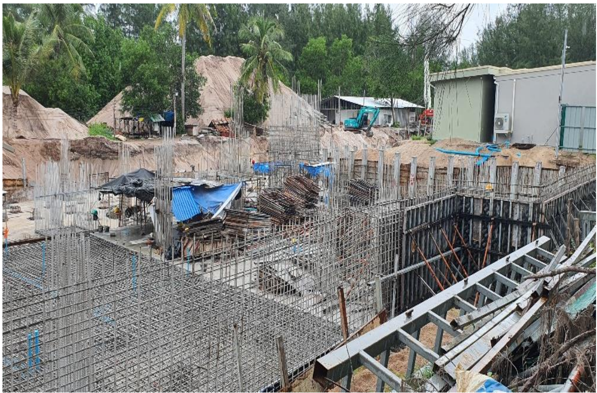
Steelwork Building 3 & Retaining wall perimeter poured building 4 – retaining wall steel in building 3 prepared ready for formwork
