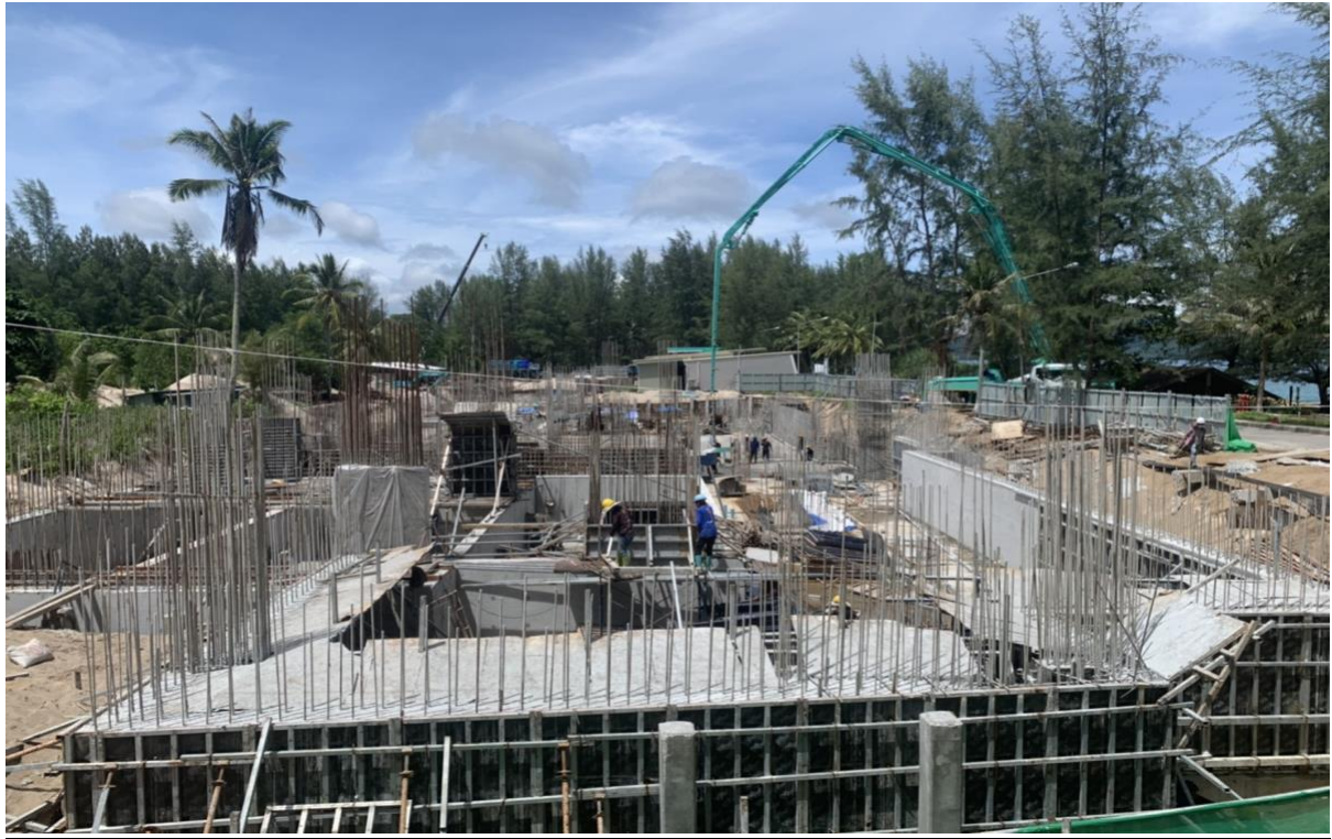
Perimeter retaining walls Emergency exit area building 1
