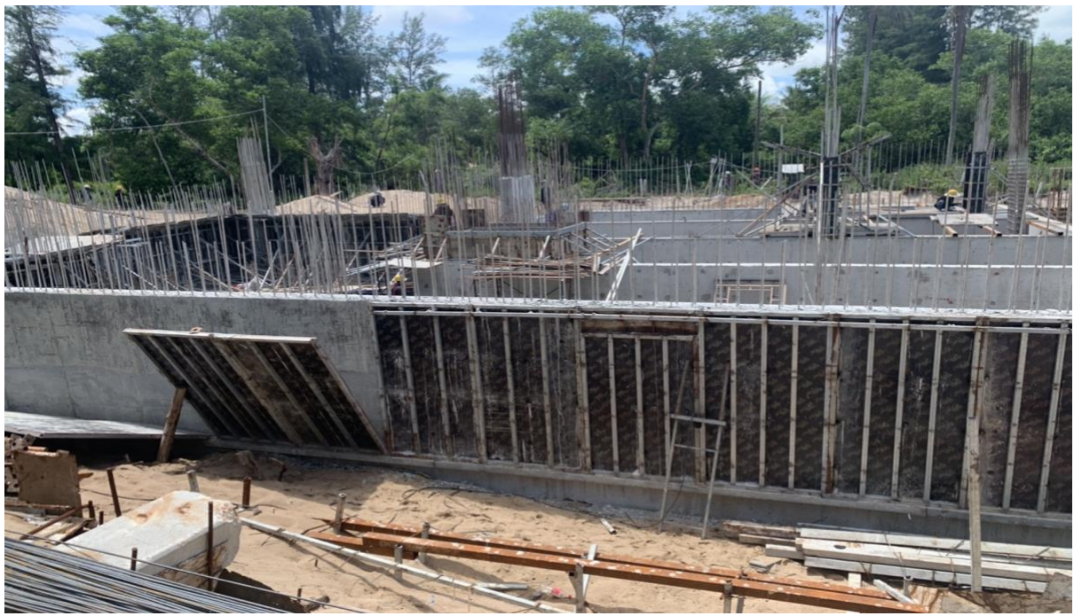
Retaining walls building 1 -Storeroom zone /Engineering Offices
