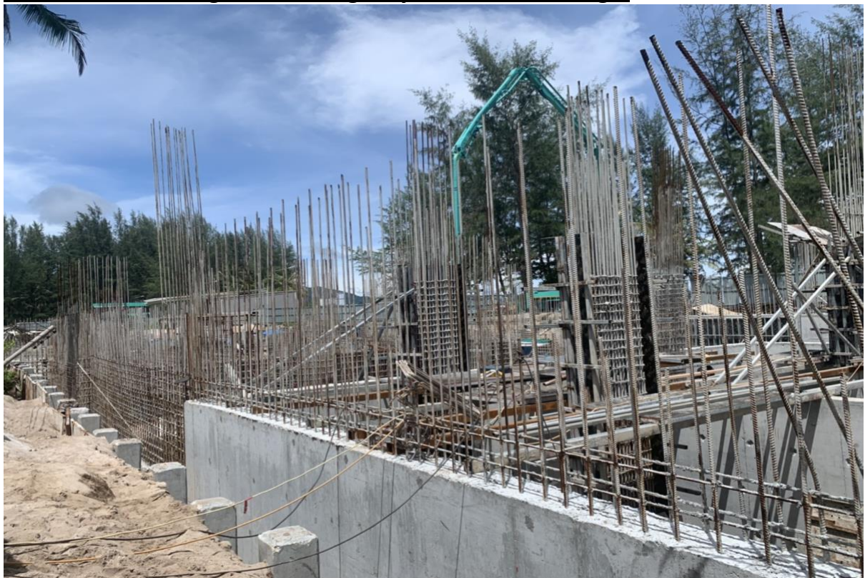
Raw tanks formwork removed/External and Internal/columns poured/commence waterproofing to enable use for storage water
