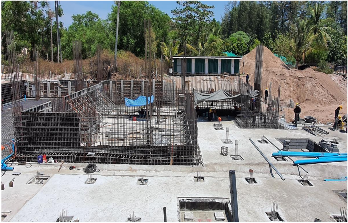
Lien in Housekeeping store & Formwork Clean Water tank Walls
