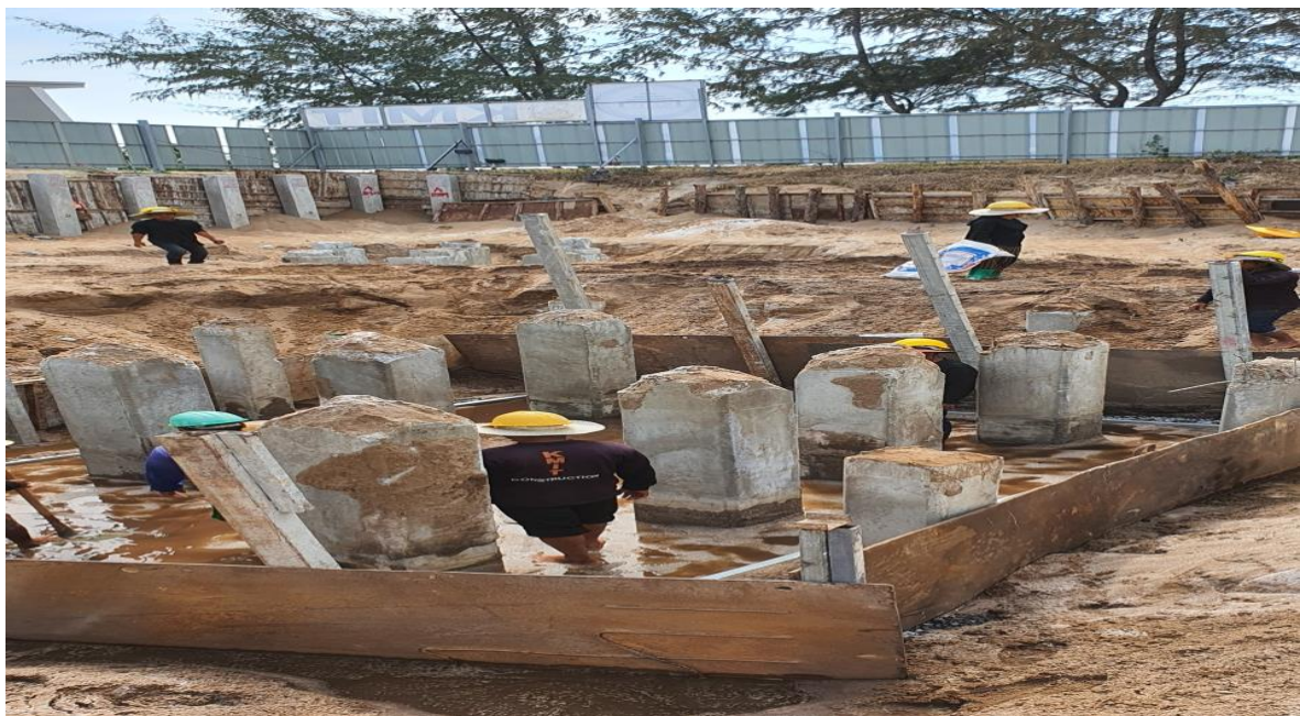
Cutting Pile heads building 3 area
