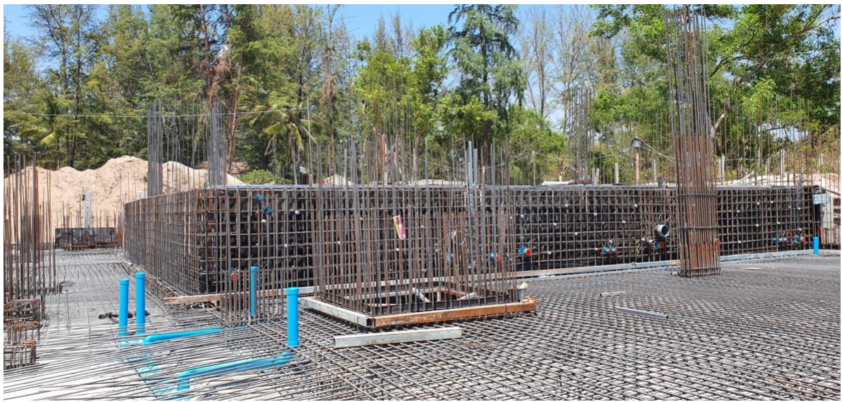
Slab preparation Pump Room & Also retaining wall formwork RAW water tanks
