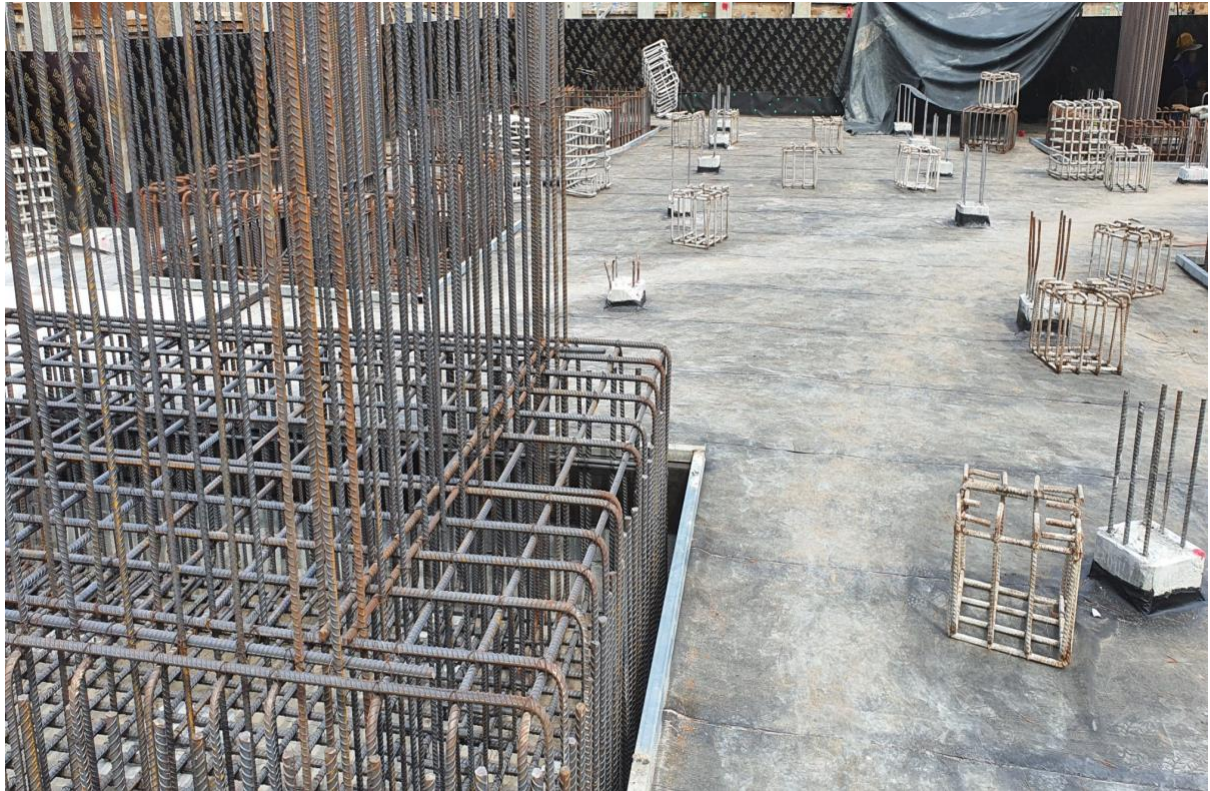
Footings and waterproofing being prepared before slab preparations
