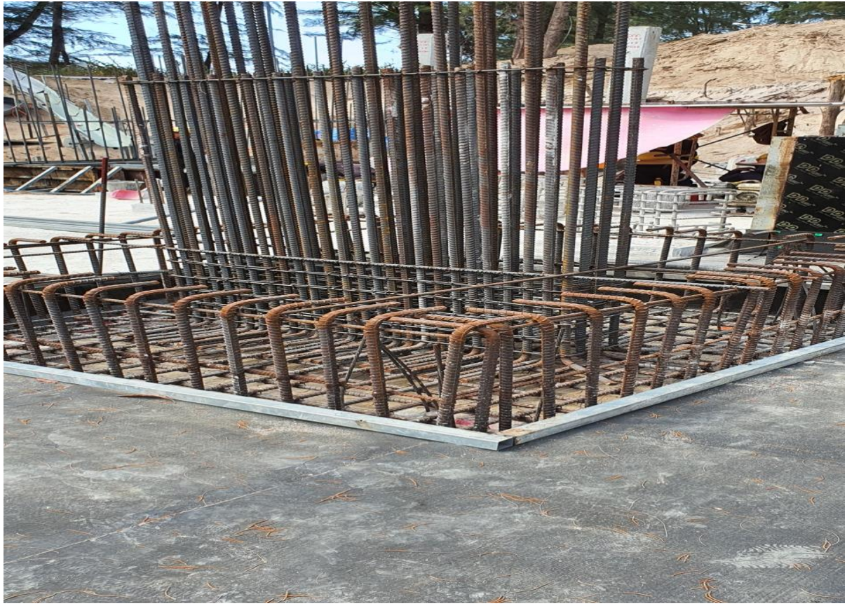
Footings and waterproof membrane preparations
