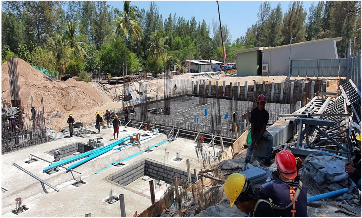
Steelwork for slab in express laundry area and Lien in Store & Corridor
