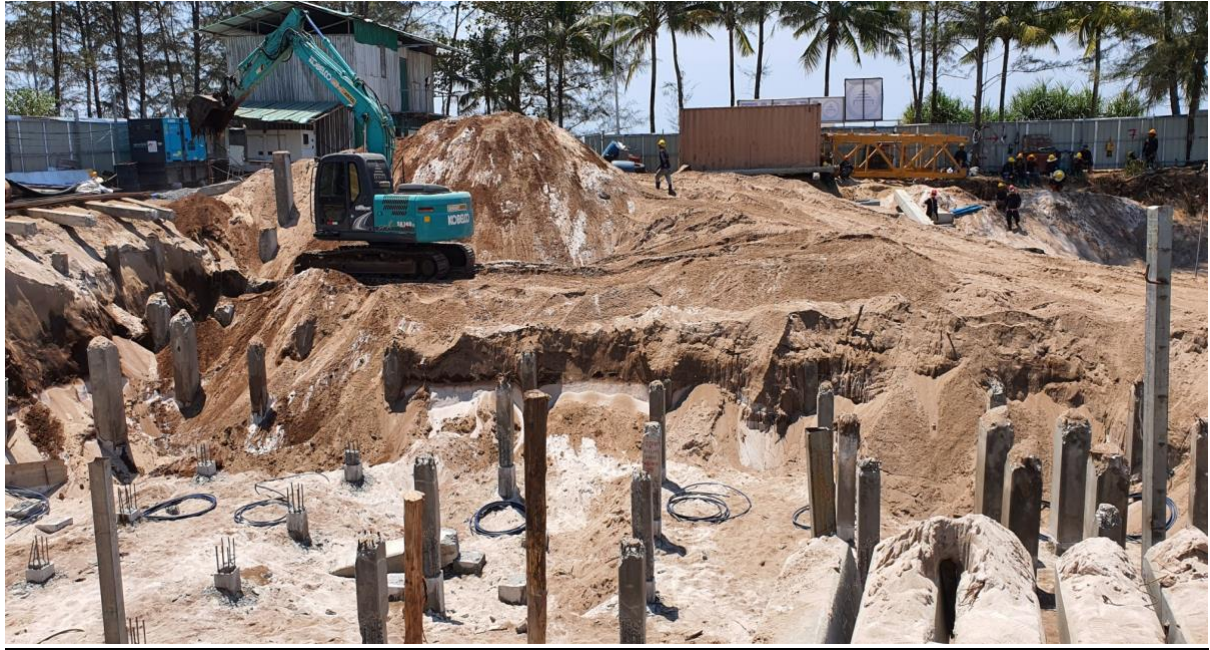
Cutting Pile Heads ready for footing in Building 8 Area
